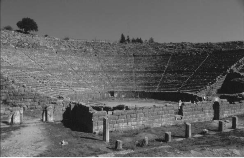
Figure 7.4 Dodona, Epeiros: the theatre constructed originally under king Pyrrhos of Epeiros (297–272 BCE) and rebuilt by Philip V of Macedon soon after 219 BCE. A building programme begun early in the fourth century, with the construction of the first temple of Zeus, culminated in the theatre. Copyright: C. B. Mee.
