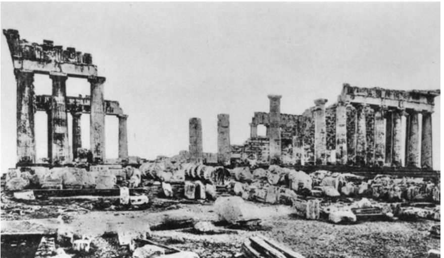
13. The transformation of the Parthenon under Balanos. His finished product (above) certainly looks more impressive than the ruin (below) from which he started. But the iron clamps used in the reconstruction soon threatened to destroy the very marble they were intended to hold together.
