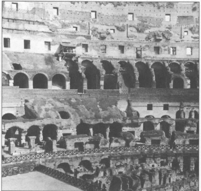
The stone seating sections were long ago removed from the interior of Rome’s greatest amphitheater, the Colosseum.
