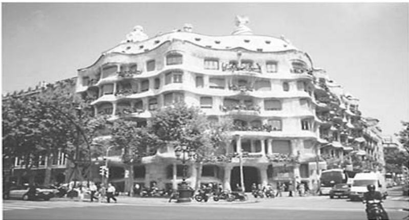
Casa Milá ("La Pedrera") (1905–10), Barcelona, Spain
