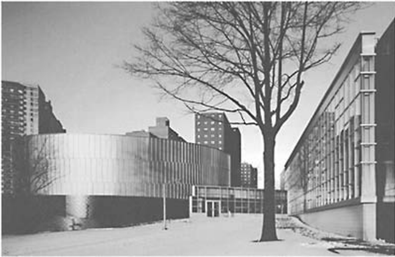
Melrose Community Center, view from south garden, Bronx, New York, designed by Agrest and Gandelsonas Architects (2000)
