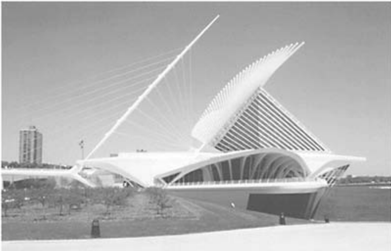
Quadracci Pavilion, Milwaukee Art Museum, South Terrace, view with wings open (2001)
