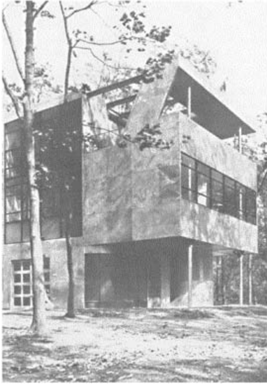
Aluminaire House, Syosset, New York, designed by Albert Frey (1931)
