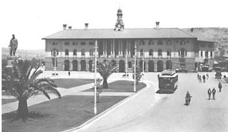
Pretoria Railway Station, Pretoria, South Africa (1909), photographed designed by Herbert Baker
