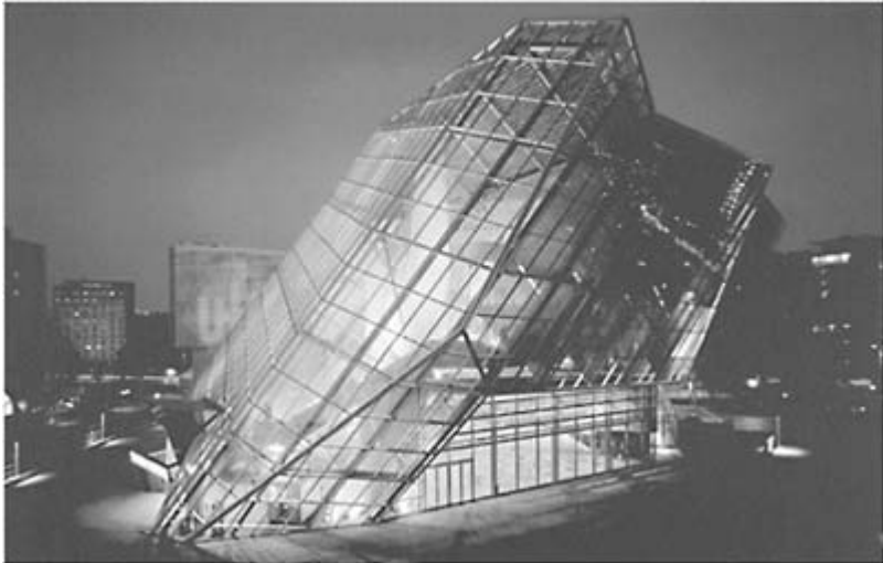
UFA Palast: Dresden, Germany (1998), designed by Coop Himmelb(l)au of Austria
