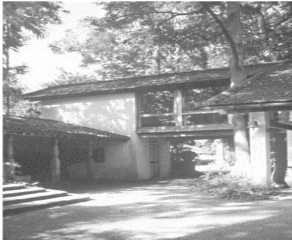
The Garden at Lunuganga, exterior view showing wood columns supporting overhang, Sri Lanka (1950), by Geoffrey Bawa
