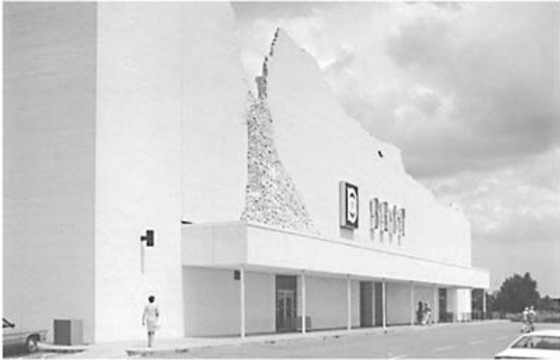
Best Products Showroom, Houston, Texas, designed by SITE (1976)
