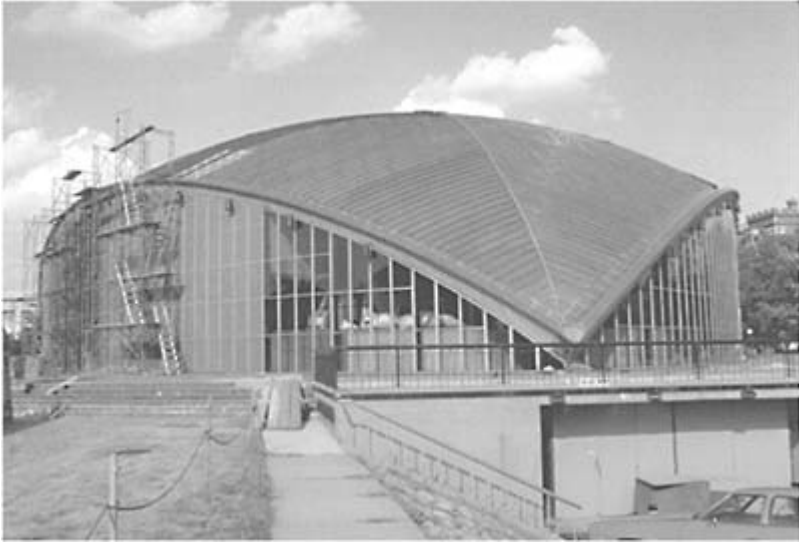
Kresge Auditorium Massachusetts Institute of Technology, shown from the rear, roof being replaced, designed by Eero Saarinen (1955)
