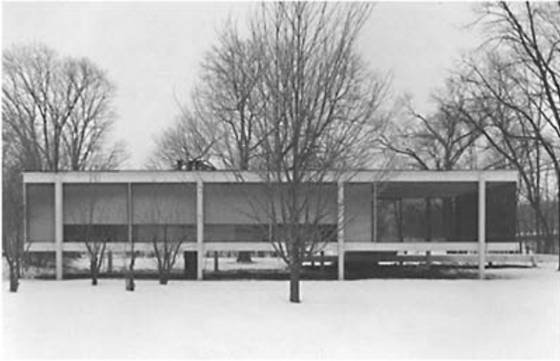
Farnsworth House, north elevation
