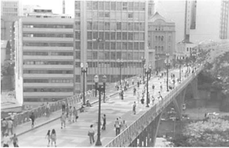
Santa Efigênia Viaduct, São Paulo, Brazil (architects unknown)
