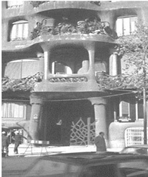
Casa Milá, close-up of entrance and balconies
