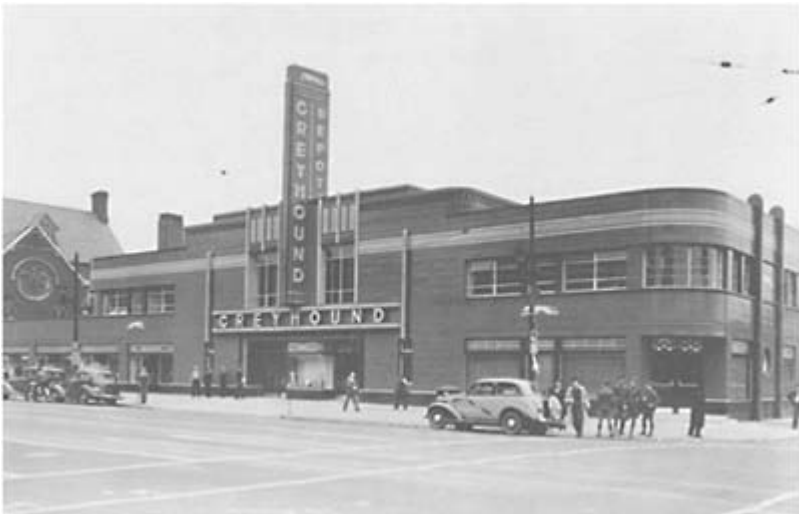
Greyhound bus station, in the streamlined art deco style, Louisville, Kentucky (1938)
