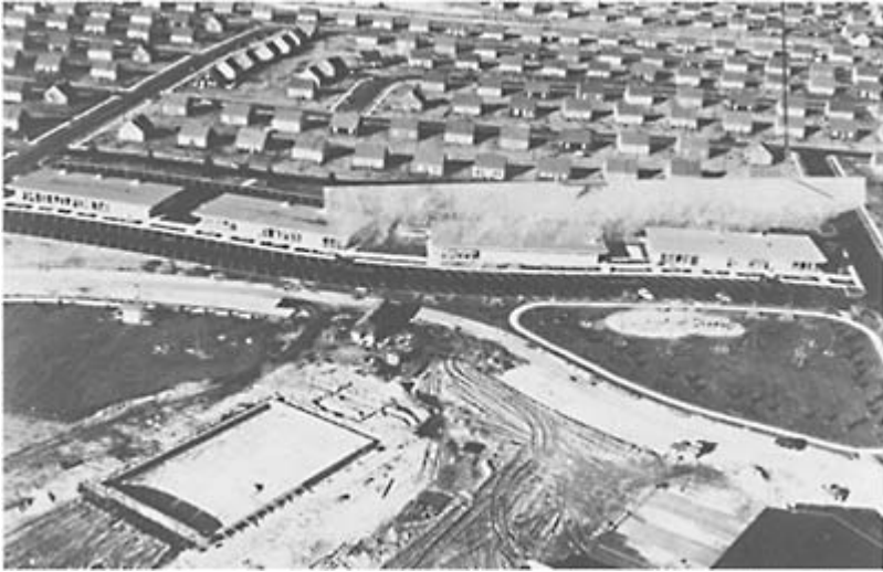
Aerial view of a housing development in Levittown, New York, under construction
