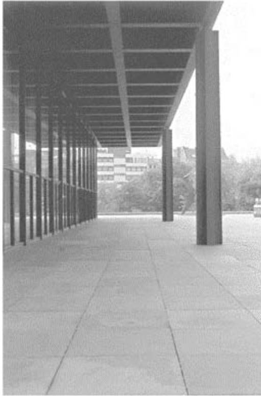
Neue Nationalgalerie, detail (New National Gallery), designed by Mies van der Rohe (1962–68)
