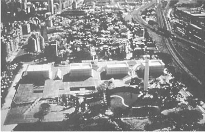
ATC (Argentina Televisora Color) Building, designed by Manteola, Sánchez Gómez, Santos, Solsona, Viñoly
