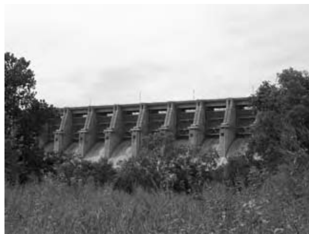
Fig. 2 Typical embankment dam in Texas, U.S.A. (View this art in color at www.dekker.com .)
