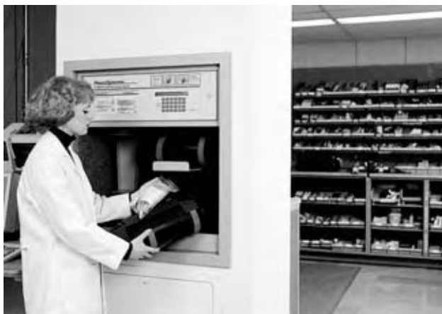
Fig. 2 Use of a computerized small PCP ("tube transport") system at the Johns Hopkins Hospital in Baltimore, MD, for transporting medical supplies. (Courtesy of PEVCO.)
