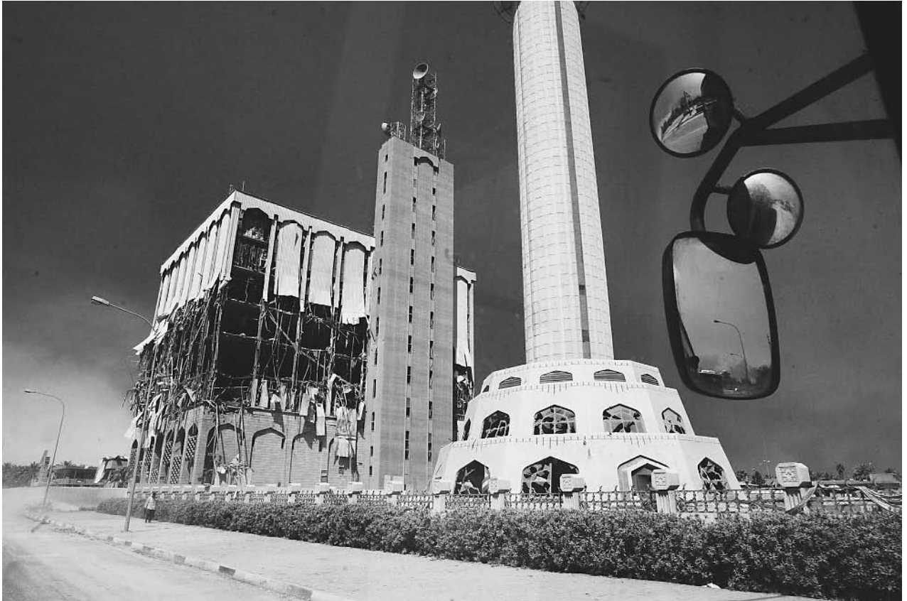
A key element of the U.S.-led coalition strategy during Operation Iraqi Freedom in 2003 was the bombing of communications centers to disrupt Iraqi intelligence as well as Iraqi command and control infrastructure. Intense bombing with precision weapons destroyed the function of this Iraqi communication building without extensive damage to surrounding buildings. AP/WIDE WORLD PHOTOS.
