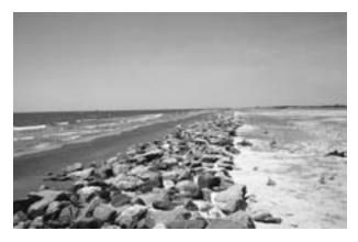
Beach protection by means of a revetment (low wall of rocks). Revetments, bulkheads, and seawalls protect the land but do not promote beach buildup. Groins and breakwaters protect the land by promoting beach buildup. *(NOAA)*
