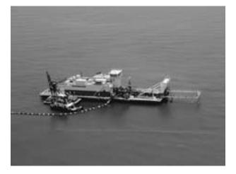
Dredges must operate frequently to establish and maintain clear and navigable channels. Dredging or the underwater excavation of channels is necessary to maintain a national system of waterways. This dredge is working in the Houston Ship Channel. (USCG-PA2 James Dillard)
