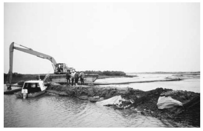
A berm being constructed for beach protection (NOAA)
