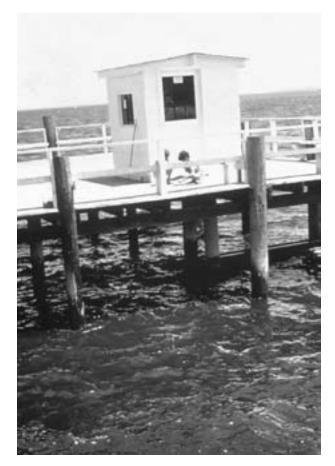
NOAA tide houses contain tide gauges, recording instruments, and possibly satellite radios. (NOAA/NOS)
