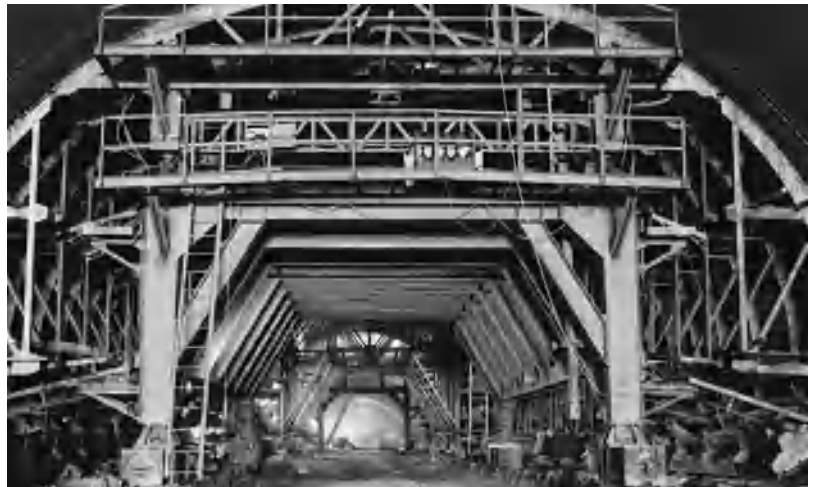
Fig. 1. Temporary supports for a four-lane road tunnel. (RESA Engineering Corporation)
