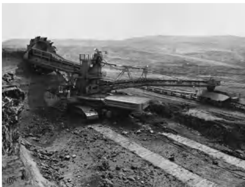
Fig. 6. Bucketwheel excavators. (a) Large type, daily capacity 144,000 yd 3 (110,000 m 3 ). (b) Smaller model.
