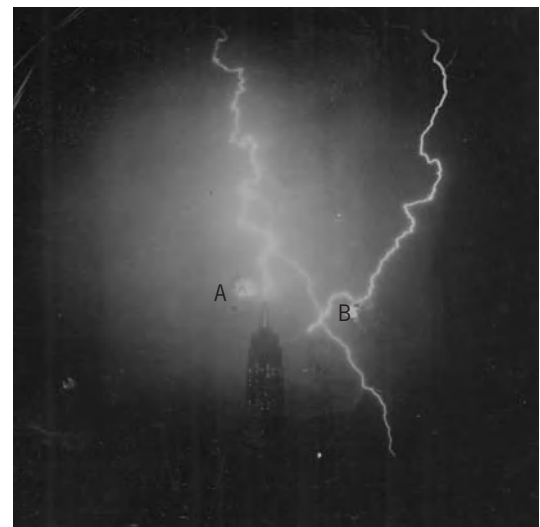
Fig. 2. Multiple lightning stroke A to Empire State and nearby buildings, August 23, 1936. Single, continuing stroke B to Empire State Building, August 24, 1936.
