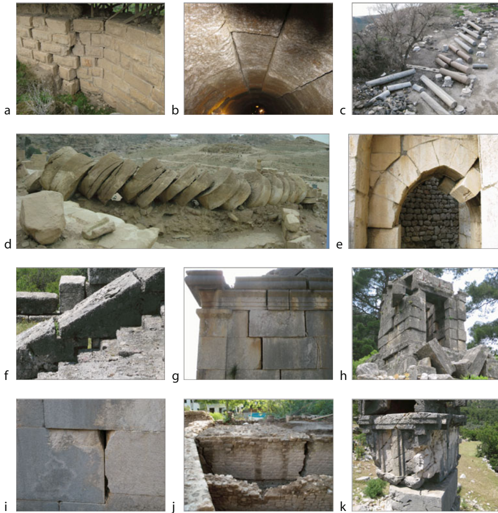
Archaeoseismology, Figure 1 Examples of deformations and damages which possibly are earthquake effects: (a) Horizontally deformed wall of a crusader fortress build on top of the Dead Sea Transform Fault in the Jordan Valley; (b) deformed vault of a Roman sewer in Cologne, Germany; (c) toppled columns of a Byzantine church in Sussita located above the Sea of Galilee; (d) toppled column of the great palace in Patra, Jordan; (e) moved block in an arch of the Nimrod fortress in the Golan Heights; (f) shifted blocks of an analemma of a Roman theatre in Pinara, SW Turkey; (g) moved blocks of a corner wall of a Roman monument in Patra, SW Turkey; (h) shifted blocks of a Roman grave house in Pinara, SW Turkey; (i) spall of block corners, same object as in (g);(j) broken and horizontally displaced fortification wall of the Roman Tolbiacum (Zülpich, Germany); (k) rotated Lycien sarcophagus in Pinara, SW Turkey.
