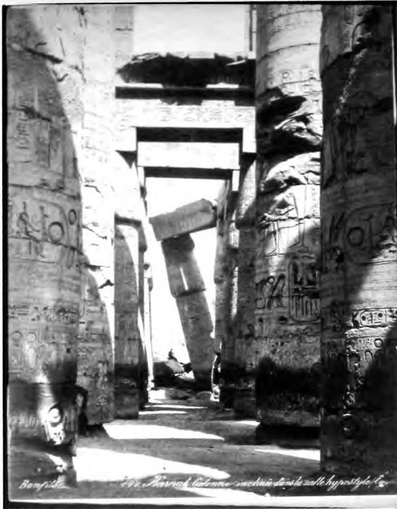
TEMPLES. Antique photograph (c.1885) of the Hypostyle Hall of the Temple of Amun at Karnak. Photograph by the Bonfils family. (University of Pennsylvania Museum, Philadelphia. Neg. # T2-988)
