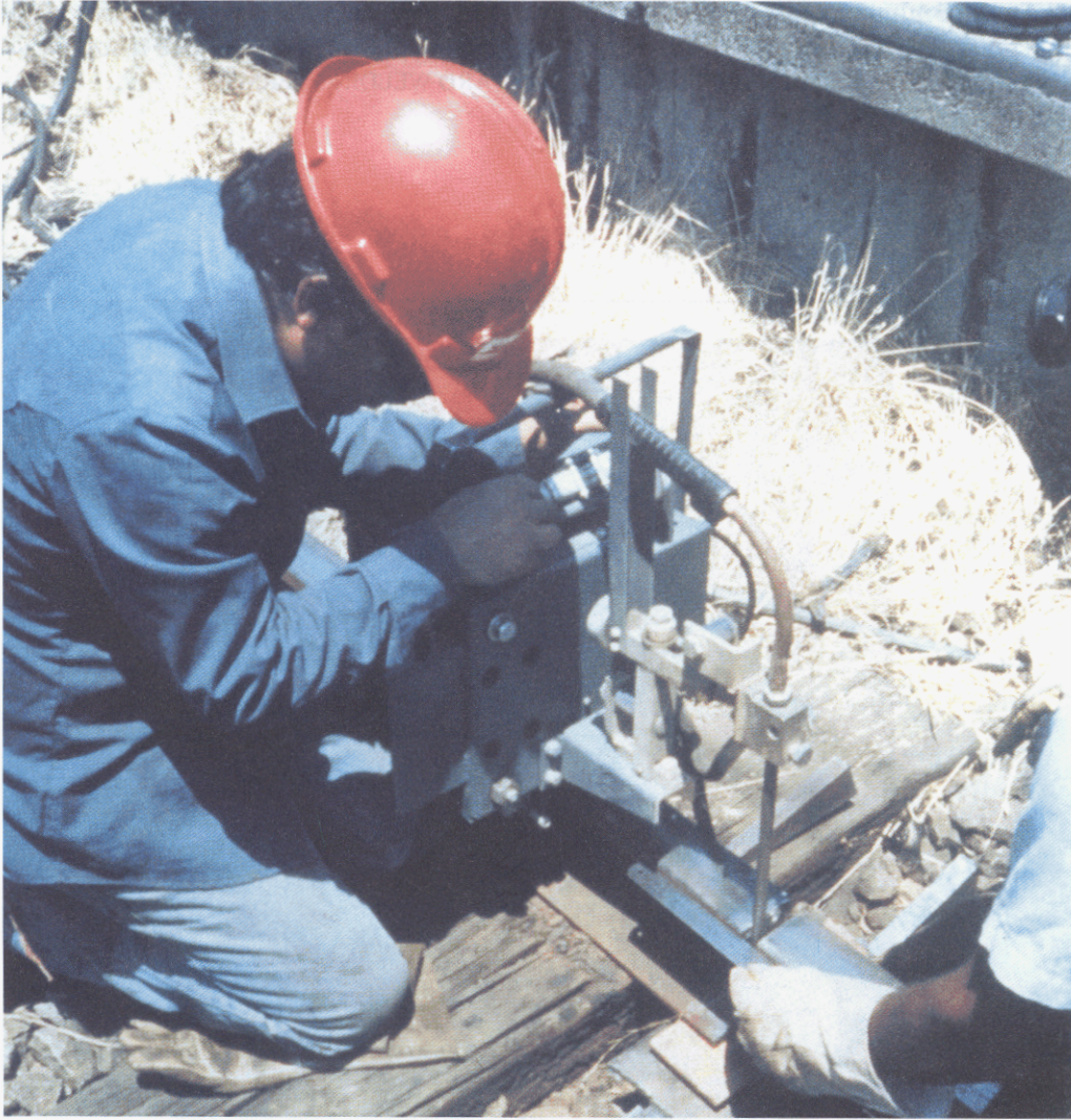
Welders set up to weld ends of rails using the electrogas process. Thermite welding is also used to provide continuous-welded railroad tracks.
