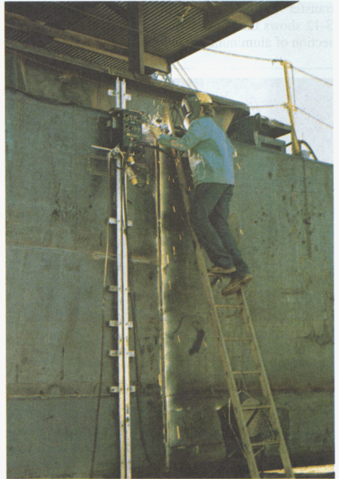
Figure S-11—Electrogas Welding of a Vertical Hull Joint
