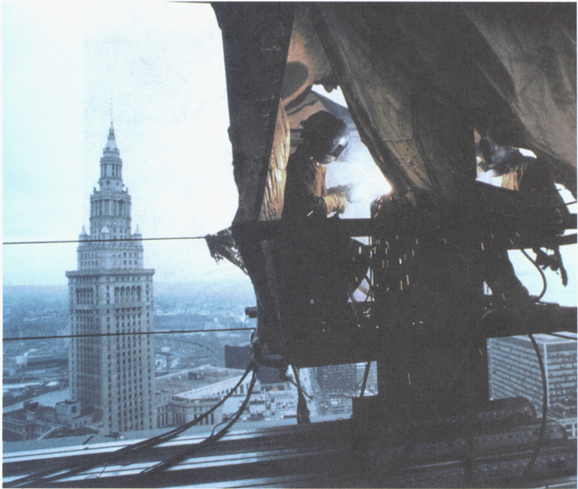
Structural Steel Welding Application BP America Building, Cleveland
