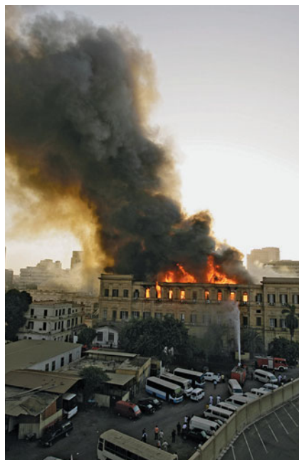
Flames and smoke rise from the People's Assembly (parliament) building in Cairo on August 19.
