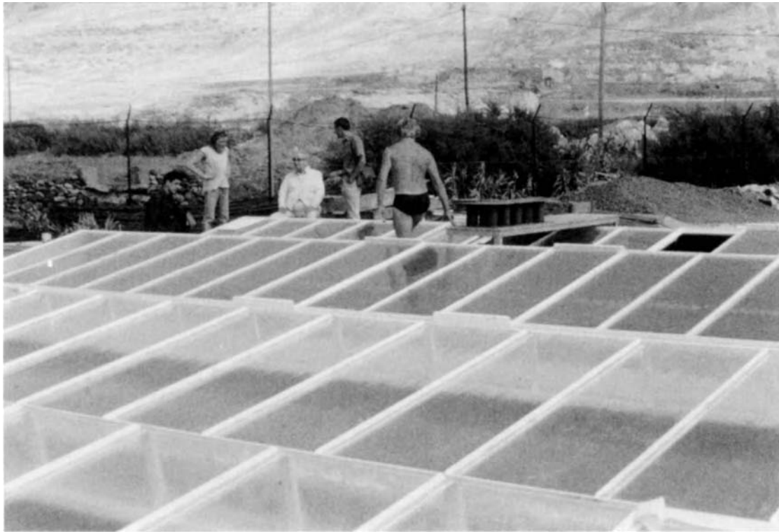
FIGURE 3 Photograph of the Solar distillation plant in Porto Santo, Madeira, Portugal. It is the only solar plant in operation in Europe. Has a total evaporating area of 1,200 m 2 , and consists from two different kinds of solar stills, of the assymetrical type. The Greek design developed at the T.U. of Athens and the design developed by the university of Berlin.
