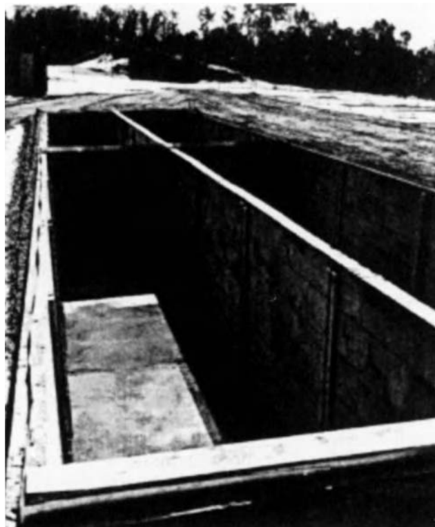
FIGURE 9 Concrete trench. Double trench, for medium-level solid wastes, is covered with a light roof when in use. The filled trench is levelled with sand and a concrete roof is poured. Note galvanized steel seals for joint.
