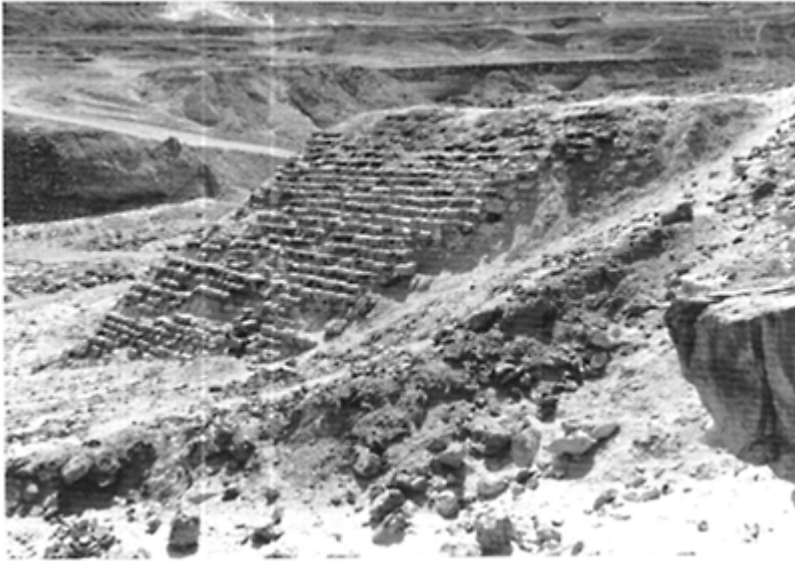
Figure 128 Upstream face of the northern wall (right bank of the wadi)
