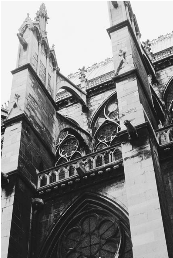
Flying buttresses, Abbey Church of St. Denis, north of Paris. The Abbot Suger began the Gothic renaissance at this abbey. (Photo by Frank K. Flinn)
