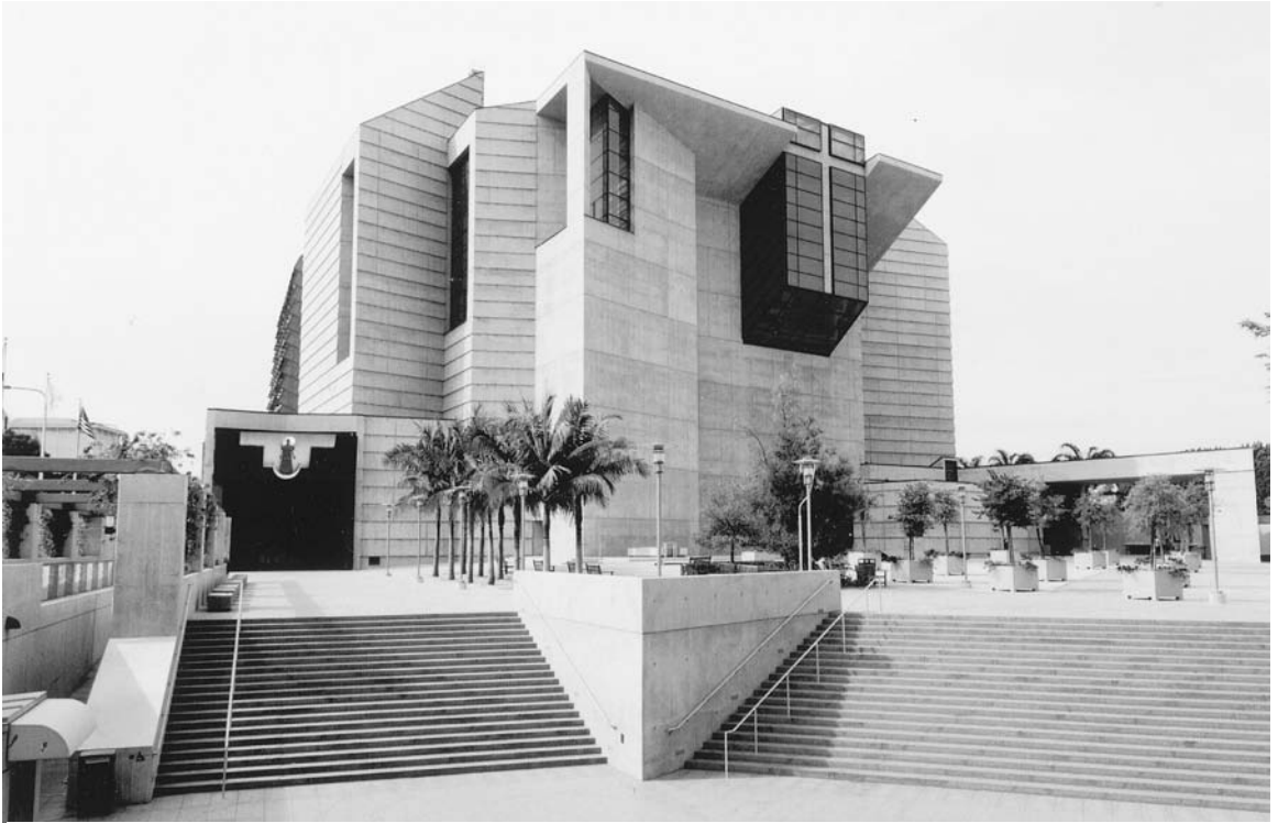
Cathedral of Our Lady of the Angels, 2002. This modernist cathedral was designed by the Spanish architect José Raphael Moneo to reflect the many-faceted cultural diversity of Los Angeles. (Los Angeles) (photo by George Machados, with permission)
