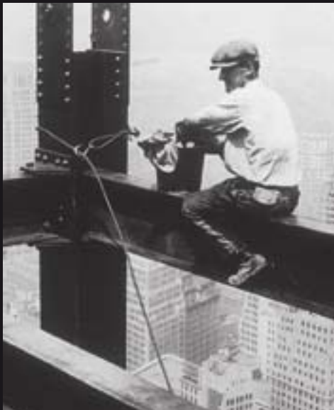
The construction of the Empire State Building in New York, USA
