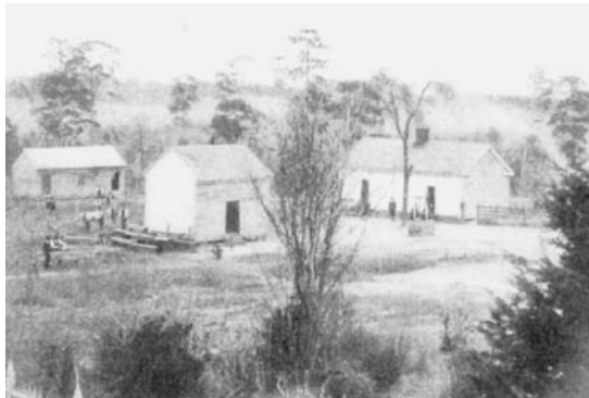
The first three buildings owned by Tuskegee. A cabin, henhouse and stable were all that remained on the plantation that Booker T. Washington purchased in Alabama in 1882 for $500 and eventually transformed into Tuskegee Institute. ( Library of Congress )
