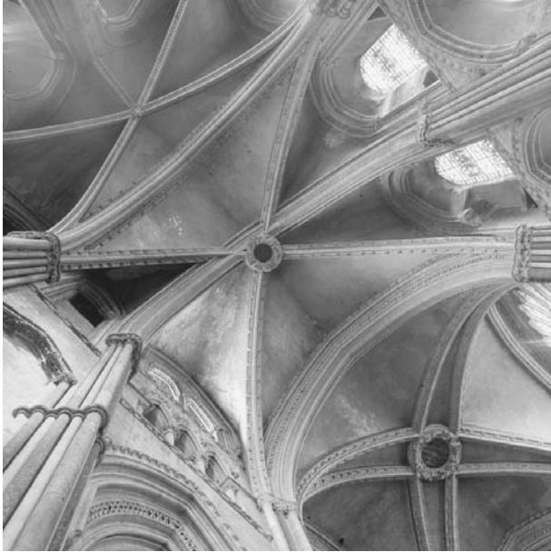
Mismatched ribbed vaulting for transept ceiling in the Chapel of the Nine Altars, Durham Cathedral, England, 1093–1133. ANGELO HORNAK/CORBIS.
