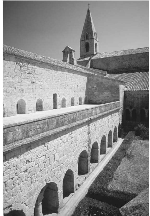
Arcaded Cloisters of Cistercian Abbey of Le Thoronet, France, late twelfth century. GAIL MOONEY/CORBIS.
