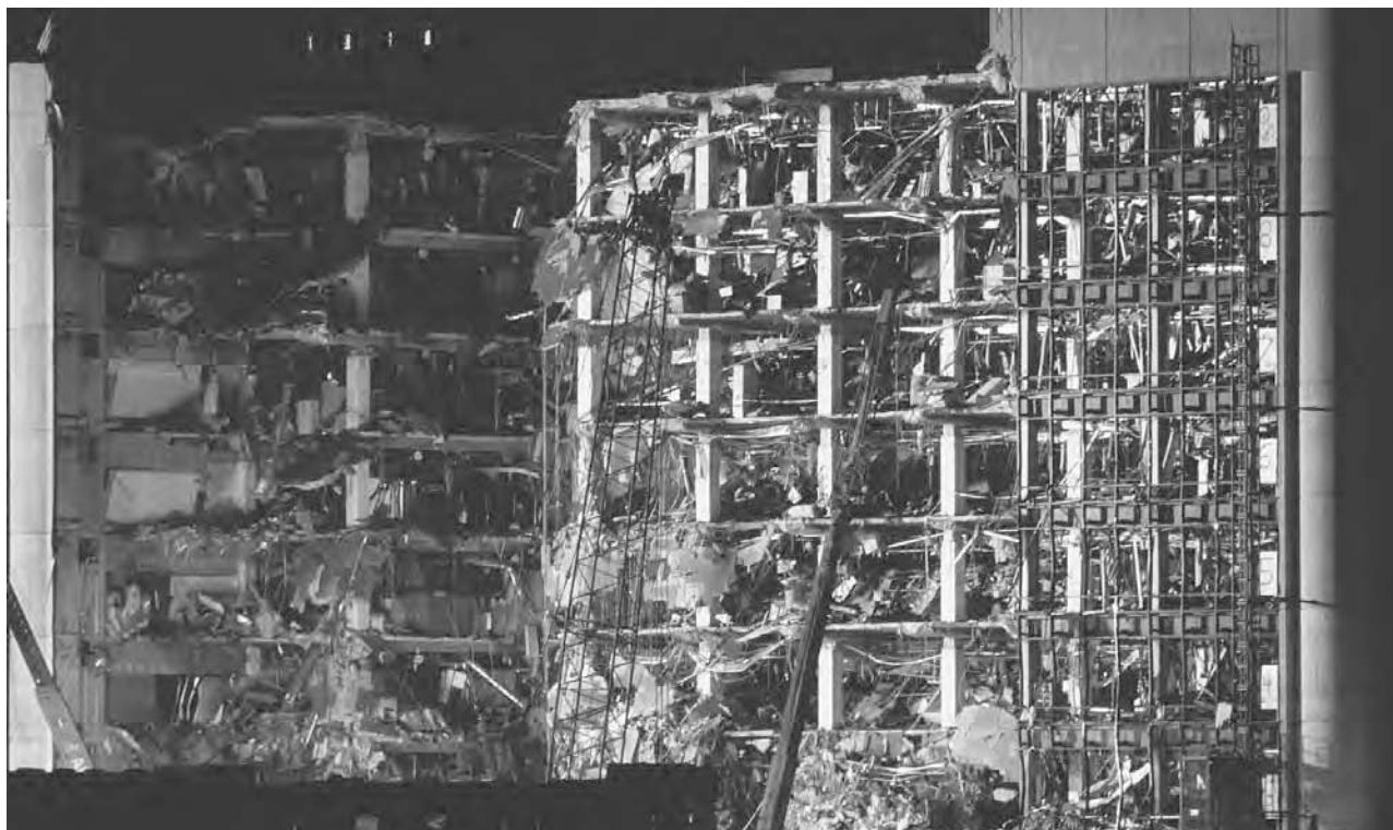
Nothing but rubble remains of the front side of the destroyed Federal Building in the Oklahoma City bombing aftermath. On 19 April 1995, a fuel-and-fertilizer truck bomb exploded in front of the Alfred P. Murrah Federal Building, killing 168 people. Timothy McVeigh was convicted on first-degree murder charges for the worst terror attack on U.S. soil up to that time. (Ralf-Finn Hestoft/CORBIS SABA)
