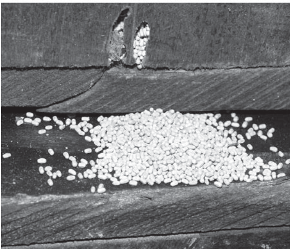
Structural Fumigation, Figure 144 Termites are the most common target pests of structural fumigation: (top) the West Indian drywood termite, Cryptoterme brevis , a widespread target of structural fumigation, (bottom) drywood termite pellets are a common sign of infestation.
