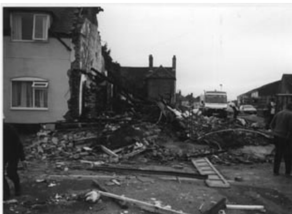
Figure 5 A typical petrol vapor explosion, which caused almost complete demolition of the building, followed by a widespread and destructive fire.
