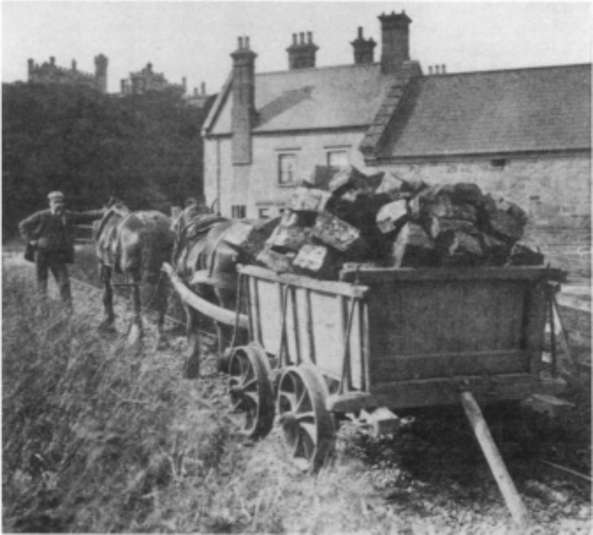
Figure 11.1: A horse railway built in 1815 to carry coal to Belvoir Castle, Leicestershire, from a canal wharf was still in use a century later. Cast-iron fish-belly edge rails can be seen.
