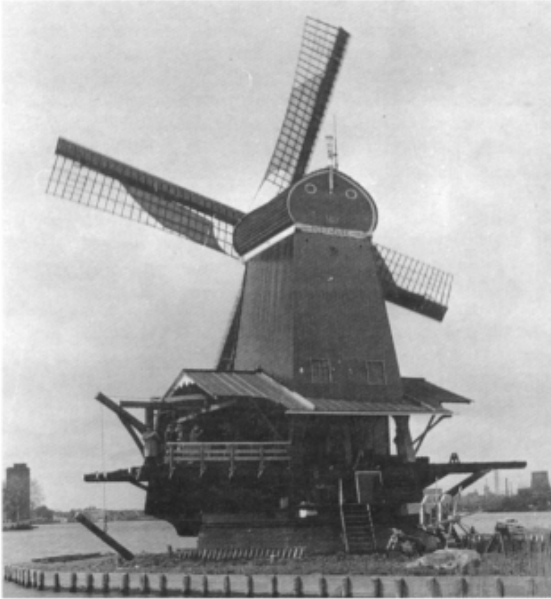
Figure 4.5: The paltrok 'De Poelenburg' at Zaandam. This saw mill was built in 1869. The brick base on which the whole mill rotates is visible behind the ladder and winding windlass. The crane for lifting the logs onto the stage is on the left. Anders Jespersen.
