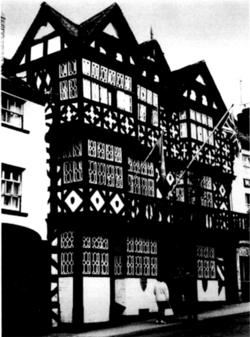
Figure 18.1: Timber-framed inn. The Feathers Hotel, Ludlow, Shropshire, late sixteenth century. Photograph Doreen Yarwood.
