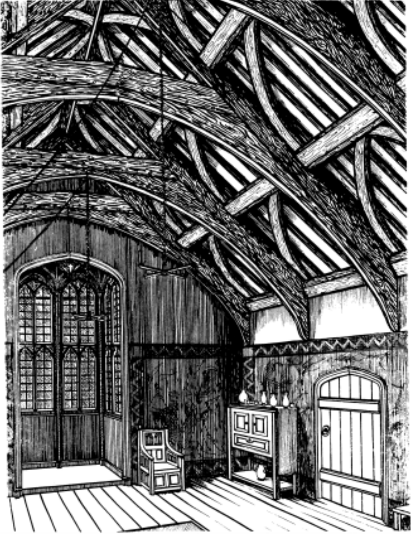
Figure 18.2: Timber-trussed roof with braced collar beams. Manor house, Solar, c. 1475–85.
