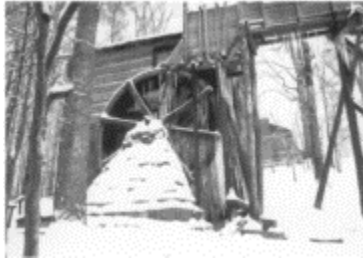
Water mill. Water flows to the water wheel along a wooden aqueduct.
