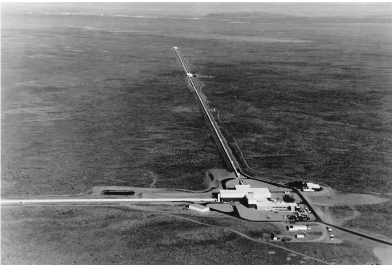
Fig. 2. Aerial photograph of the LIGO at Hanford, Washington. This facility houses two interferometers (a nearly identical facility, with a single interferometer, is in Livingston, Louisiana). The lasers and optics are contained in the white buildings; the 4-km-long (2.5-mi) vacuum tubes are covered by the arched concrete enclosure.
