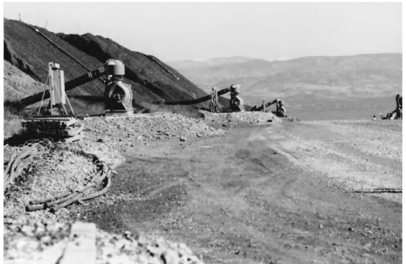
Fig. 2. Forced-air ventilation of sulfide ore heaps during biooxidation.
