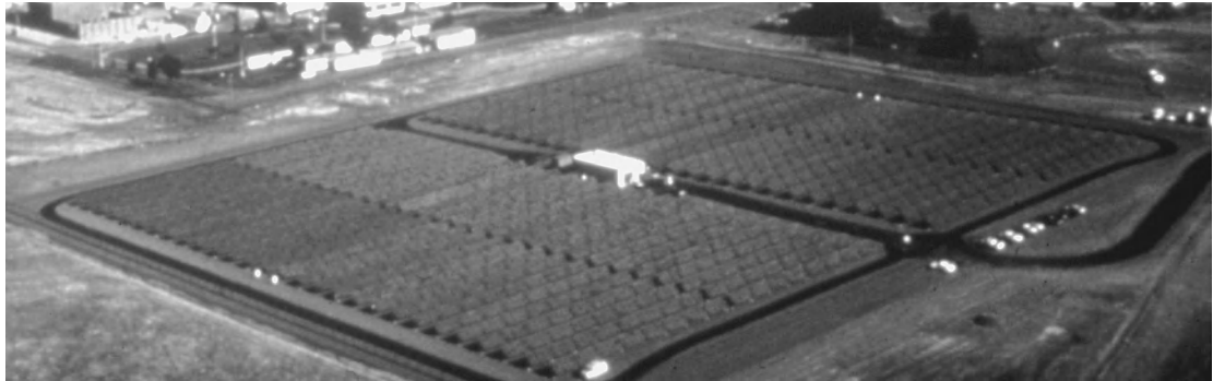
Fig. 3. A 2-MW photovoltaic array. (Sacramento Municipal Utility District, California)
