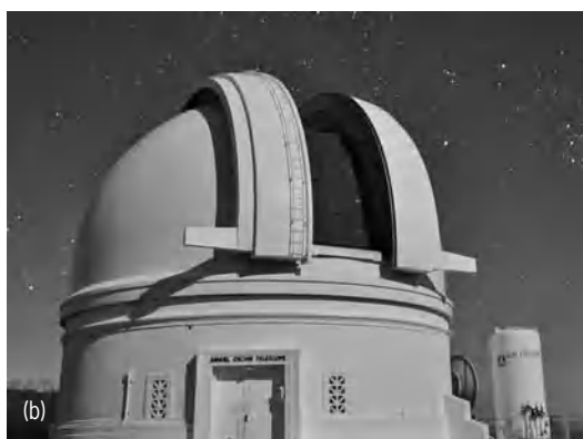
Fig. 2. Samuel Oschin Telescope, a 48-in. (1.2-m) Schmidt camera at Palomar Observatory. (a) Interior view (Alain Maury). (b) Exterior view. A large liquid nitrogen tank to the right of the open dome is used for cooling the instrument. (Scott Kardel)
