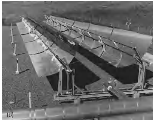
Fig. 6. Parabolic trough system. (a) Schematic of the components (after Jet Propulsion Laboratory, Fact Sheet on Parabolic Trough Systems: A Solar Thermal Concentrating Collector Concept , 5106-22/3, 1982). (b) Typical system (Solar Energy Research Institute).
