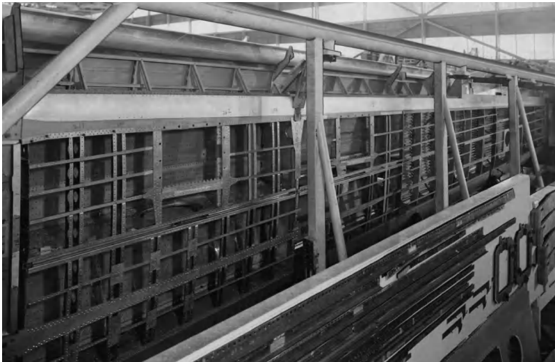
Fig. 15. Lower surface framework of outer wing of a commercial transport.
