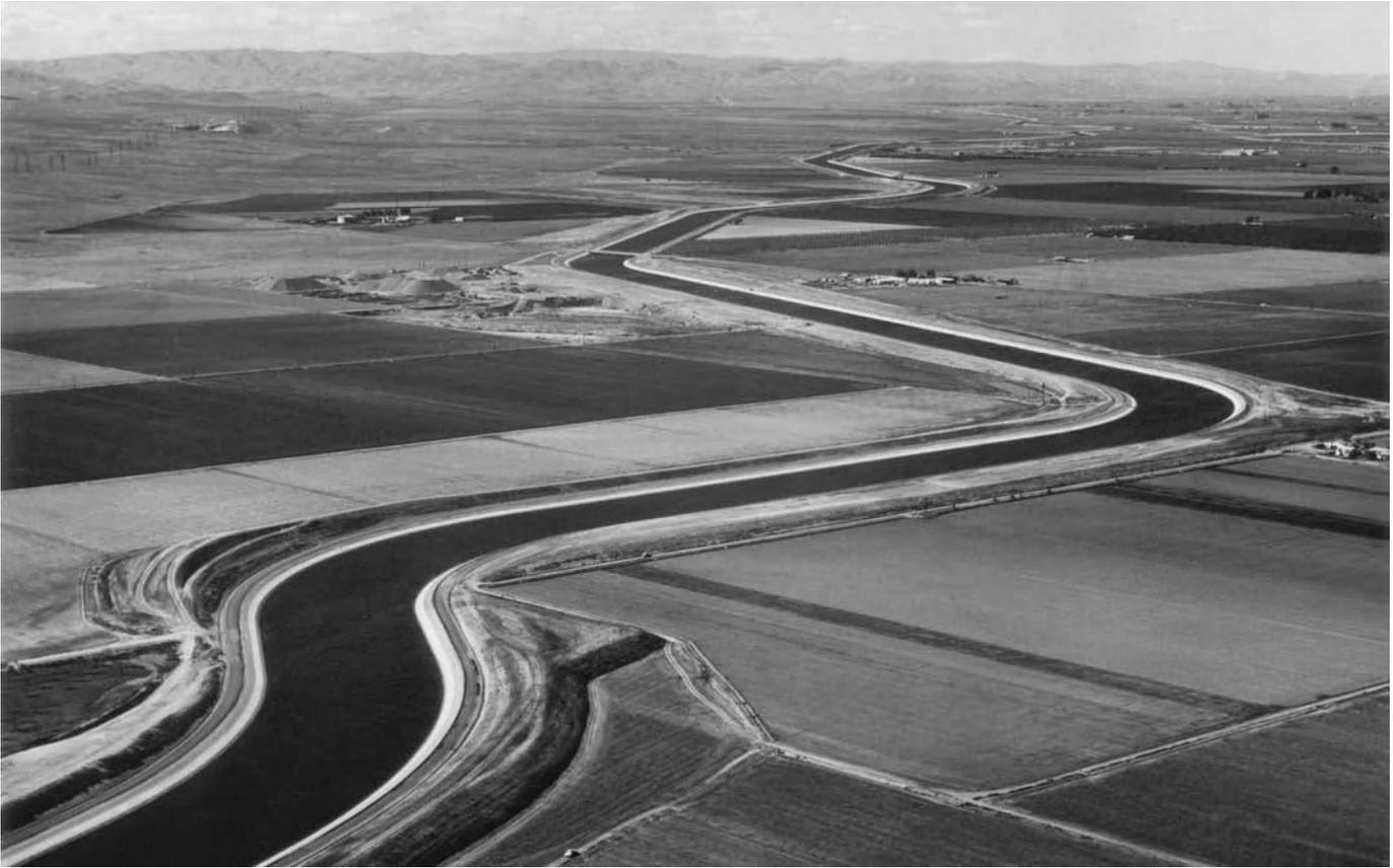
Fig. 1. Segment of the San Luis irrigation canal in California. A major waterway in the western United States, it is 103 mi (165 km) long, 200 ft (60 m) wide, and 36 ft (11 m) deep. (U.S. Bureau of Reclamation and State of California)
