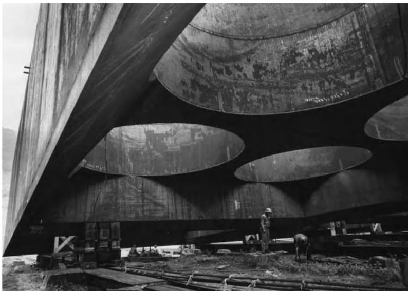
Fig. 1. Underside of open caisson for Greater New Orleans bridge over Mississippi River. (Dravo Corp.)
