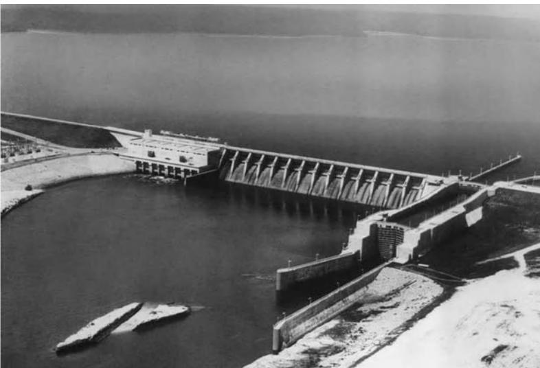
Fig. 2. Walter F. George Lock, Dam and Powerhouse on the Chattahoochee River, Alabama-Georgia boundary. The lock chamber can be seen at right center of the photograph. (U.S. Army Corps of Engineers)
