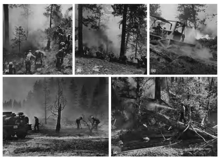
Fig. 6. Land fire suppression methods. (a) Digging a trench ahead of an approaching fire. (b) Constructing a fire line to stop the advancing fire. (c) Bulldozer making fire lane near the edge of the fire. (d) Using a tank truck to suppress fire. (e) Fighting fire with hose attached to a portable pump. (U.S. Forest Service)
