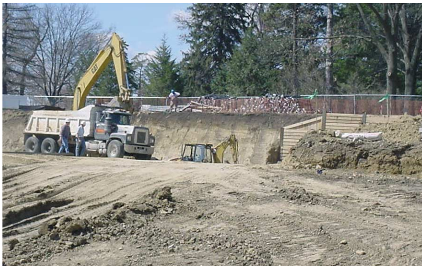
Figure 4 Urban soil being created after the natural soil has been removed. Note natural soil profile in background. Photo by Julie McLaughlin.
