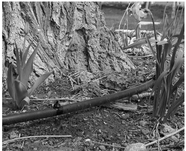
Figure 6 Pressure-compensating drip emitter watering ornamental plants.
