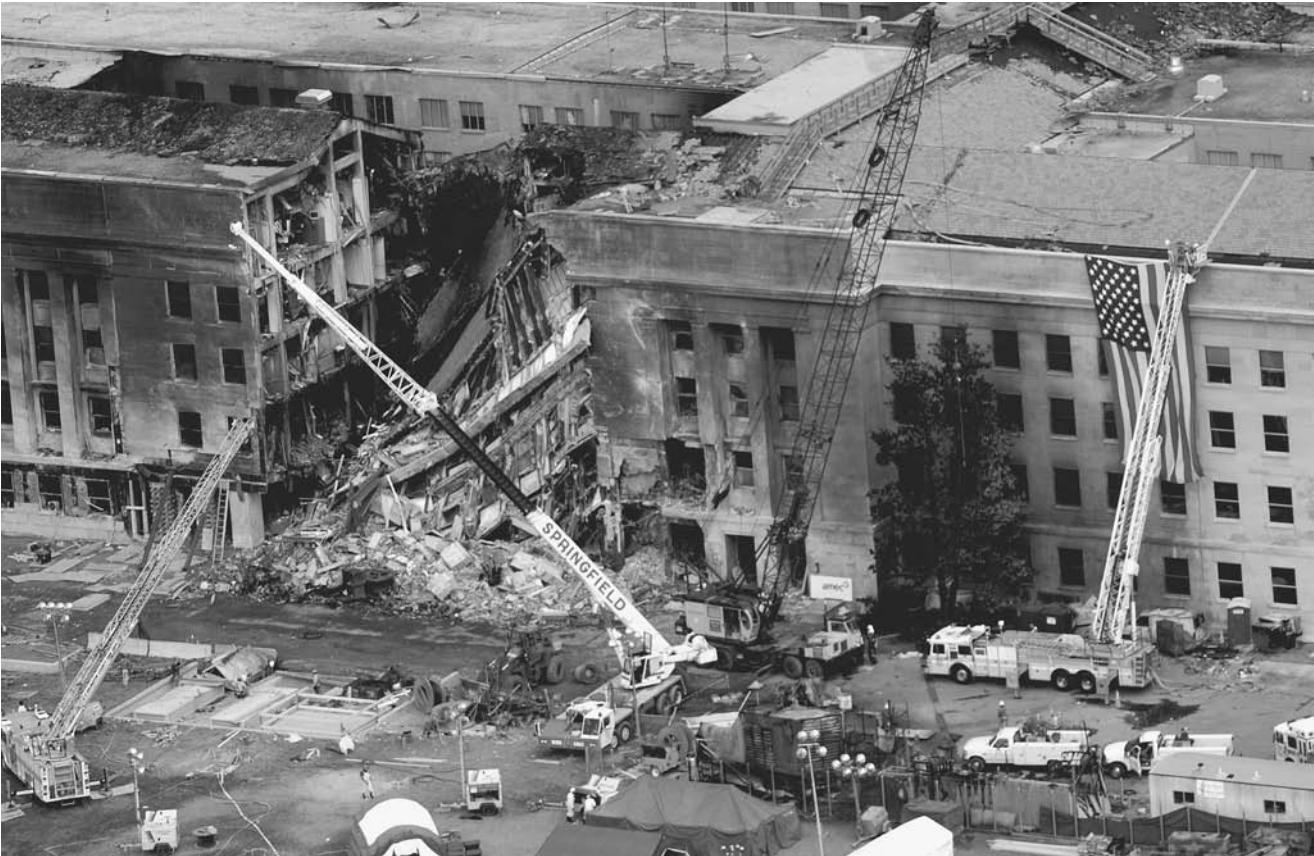
Firefighters, rescue workers, and engineers work at the Pentagon crash site on September 14, 2001.
