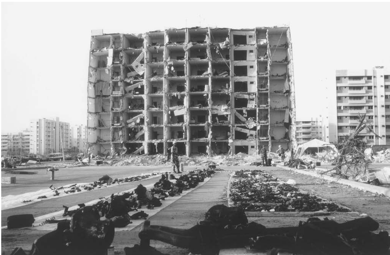
Khobar Towers, Saudi Arabia, after the 1996 bombing of the high-rise barracks that killed 19 U.S. soldiers.
