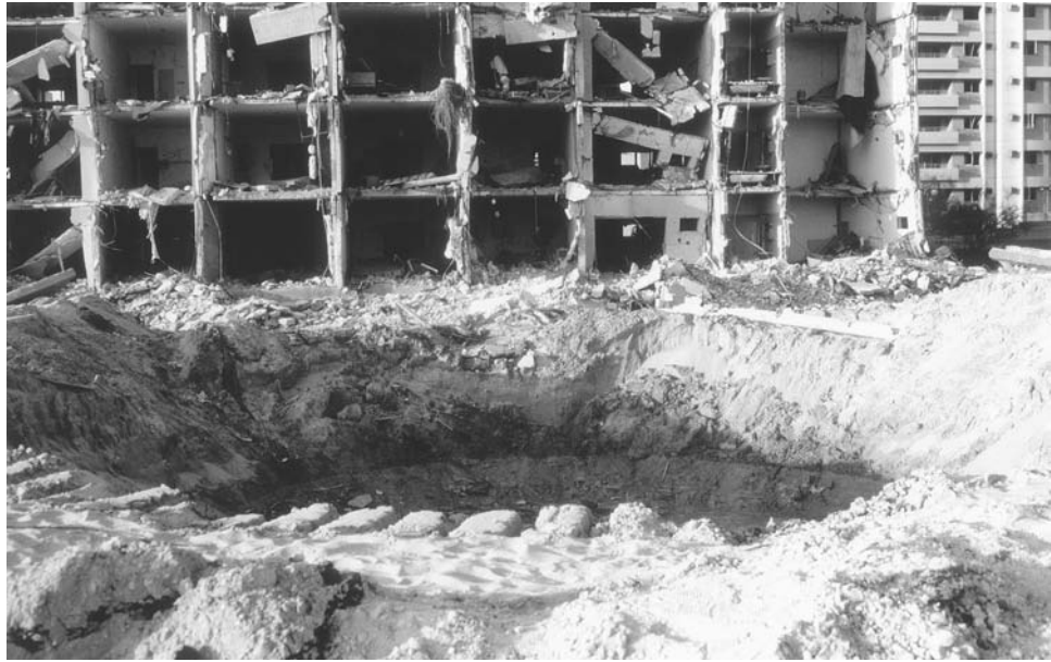
The bomb crater in front of the severely damaged north side of the Khobar Towers complex. The explosion of a fuel truck set off by terrorists on June 25, 1996, killed 19 and injured hundreds.
