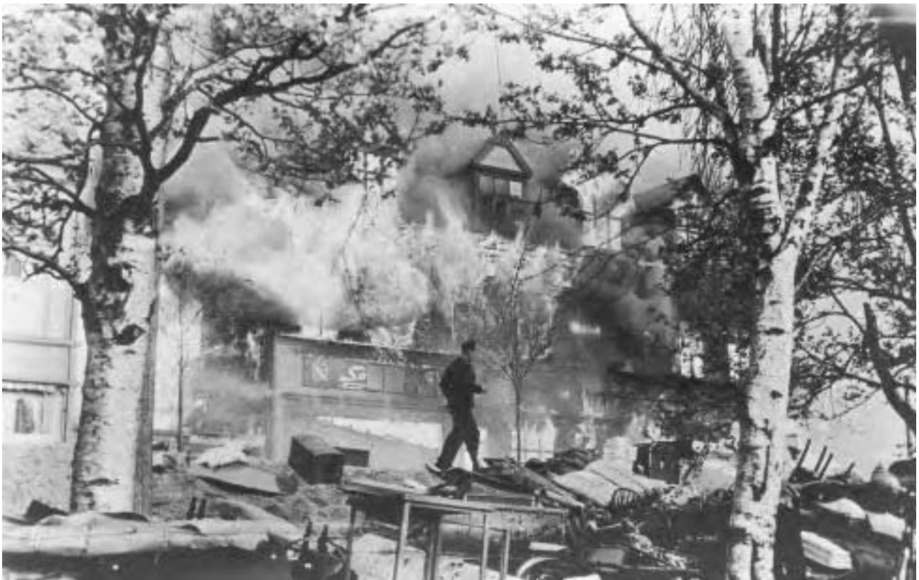
A man runs through wreckage in front of a large house in flames, following Luftwaffe air raids during the German occupation of Narvik, Norway, 2 June 1940. (Photo by R. Gates/Hulton Archive/Getty Images)
