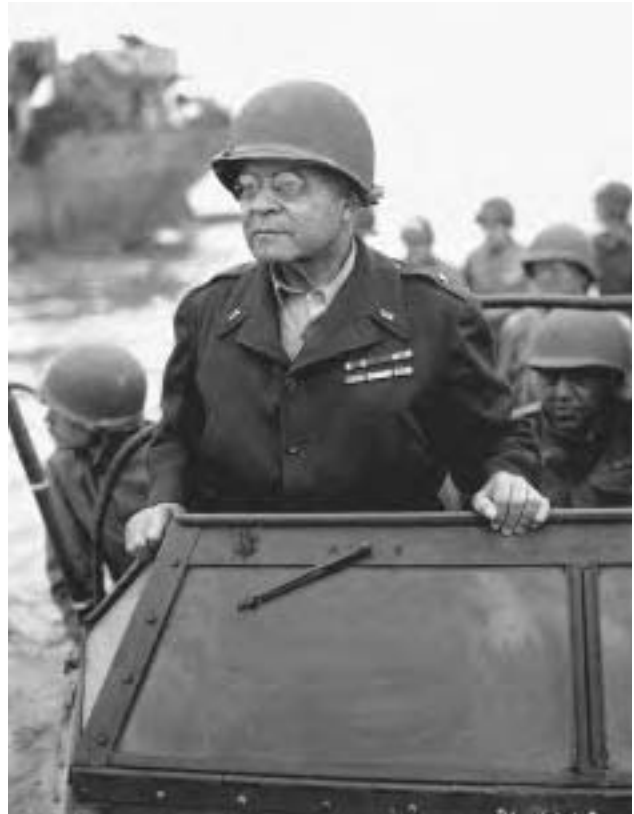
Brigadier General Benjamin O. Davis Sr. watches a Signal Corps crew erect poles in France, 8 August 1944. (National Archives)
