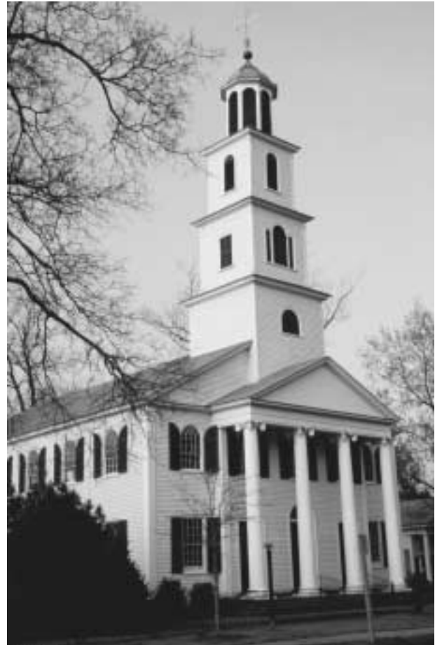
First Presbyterian Church in New Bern, North Carolina.
