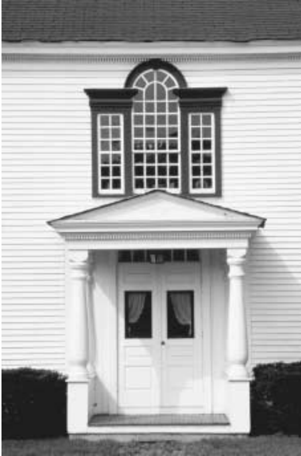
Nathan Smith House. The Palladian window and portico entry of the Nathan Smith house, built in 1791 in Cornish, New Hampshire, were characteristic of Federal or Adam style, and stood in contrast to the often-unadorned entrances of Georgian homes. © LEE SNIDER/PHOTO IMAGES/CORBIS.
