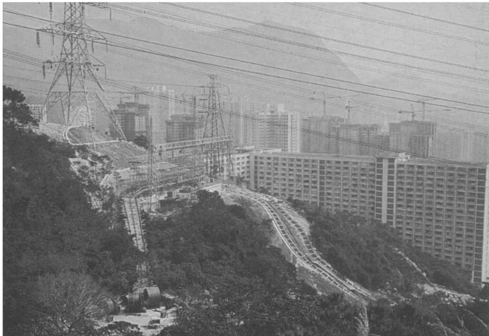
Fig. 36.3 A bond pull route for 400 kV PPL cable which has a very steep gradient in addition to onerous bends at termination positions
