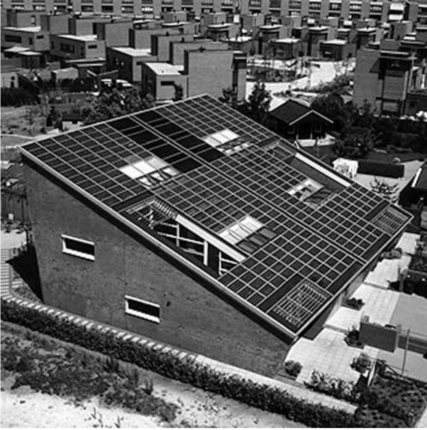
FIGURE 2.3 Roof-mounted Dutch PV subdivision, Nieuwland, in Amersfoort.
