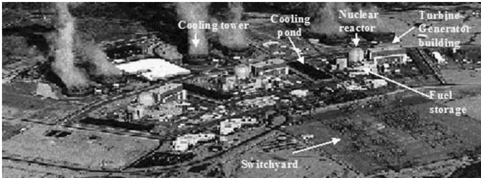
FIGURE 1.13 View of Palo Verde nuclear power plant. (Courtesy of Salt River Project.)
