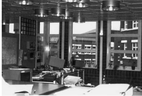
FIGURE 12.26 The Colonia Headquarters Has a Modular Reconfigurable Ceiling with Plug-and-Play Capability for Relocating Light Fixtures with Each Workstation Layout Change (ABSIC; Germany, 1989).
