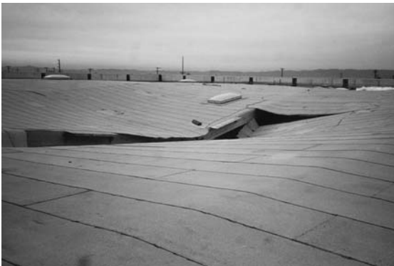
FIGURE 7.4 Heavy Snow Loads Allowed to Build on the Roof Can Lead to a Structural Collapse.
