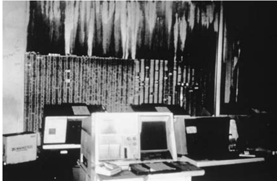
FIGURE 7.9 If Untreated, Electronics Exposed to Heavy Concentrations of Acidic Soot Will Be Ruined within Hours.
