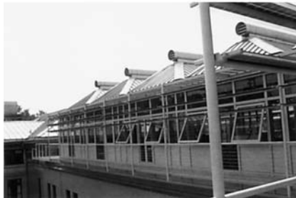
FIGURE 12.19 The Robert L. Preger Intelligent Workplace Demonstrates A Layered Enclosure, with Dynamic Light-Redirection Louvers, Operable Windows, High-Visibility Glass, and Internal Shading Devices, To Maximize Daylighting and Solar Control As Well As Support Natural Ventilation (Façade engineered, manufactured, and donated by Josef Gartner & Company).
