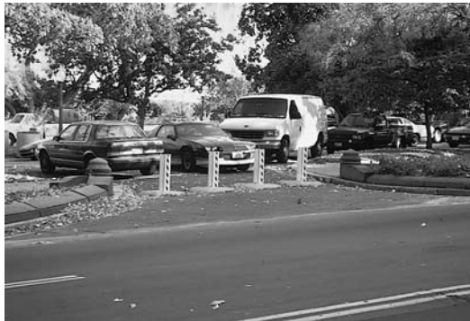
FIGURE 24.1 Vehicle Barriers (Bollards); U.S. Capitol Grounds.
