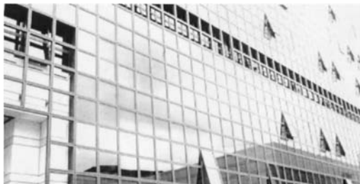
FIGURE 12.10 In the Ministry of Finance in Paris, Operable Windows Provide Occupants with Outside Air As Desired, but Avoid Energy Waste by Shutting Off the Perimeter Heating/Cooling Unit (ABSIC; France, 1991).
