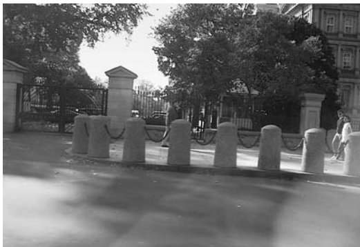
FIGURE 24.3 Vehicle Barriers (Concrete Bollards); The White House.
