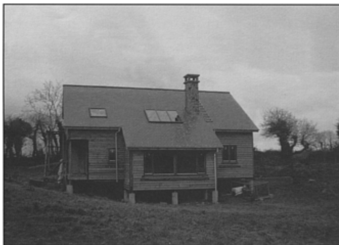
Plate 10. House in Sligo, Republic of Ireland
