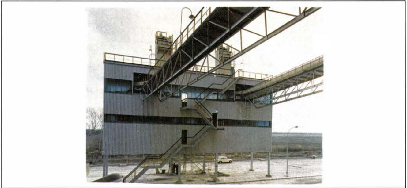
Plate 15.8 Loading station for bulk dispatches of clinker.
