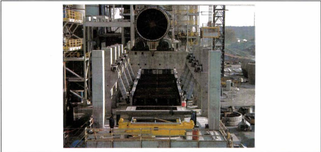
Plate 11.3 Pendulum cooler under installation.
