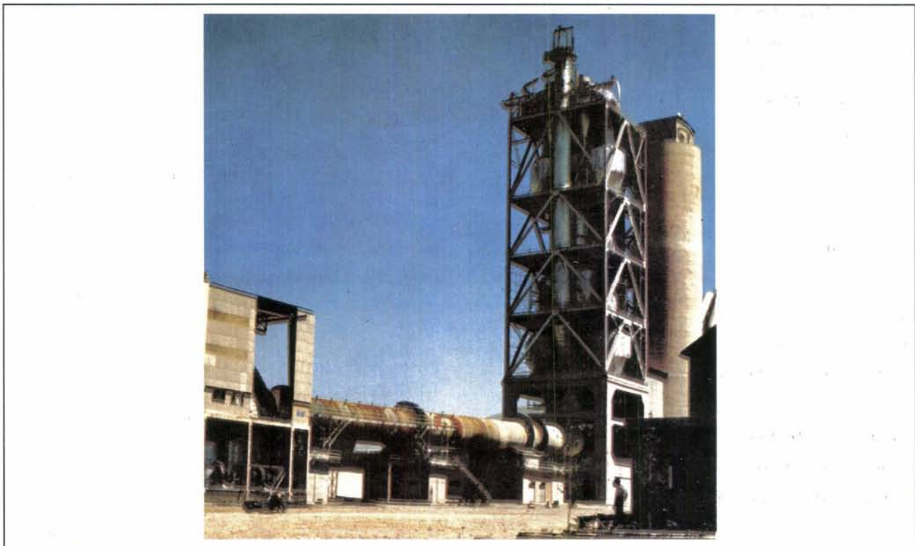
Plate 10.2 Dry process rotary kiln with preheater and grate cooler.
