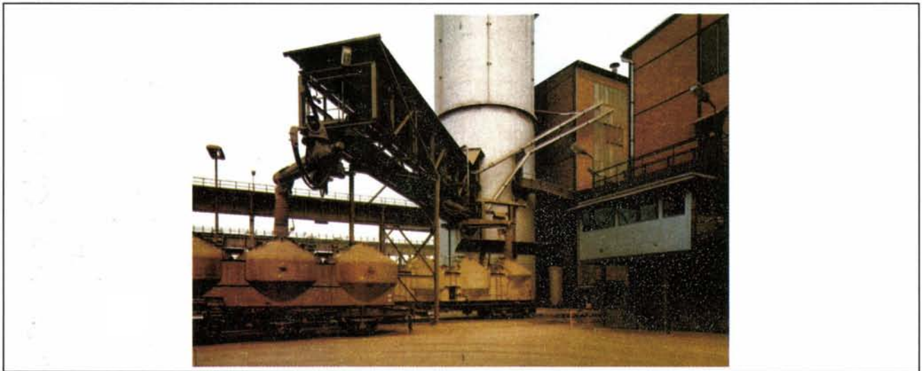
Plate 15.9 Loading bulk carriers for rail transport of cement/fly ash.
