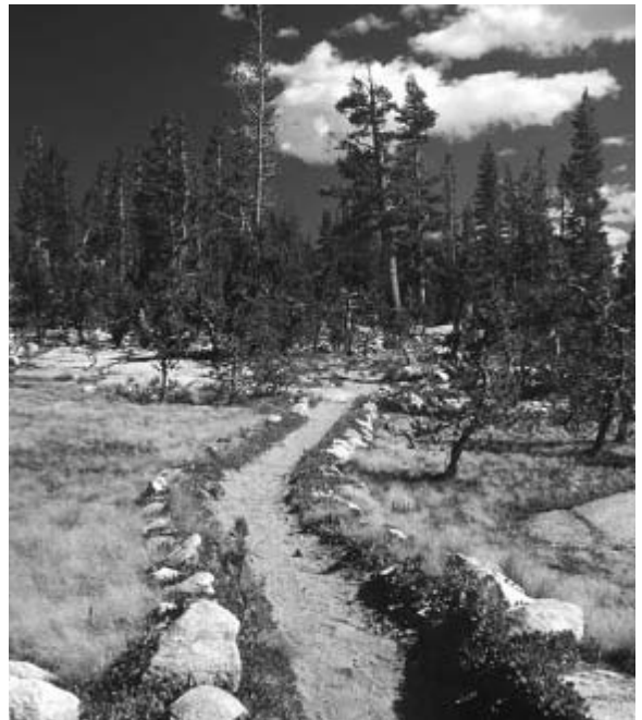
Top: A well-constructed mountain trail. The John Muir Trail below Selden Pass. Note the rocks lining the trail to keep it in place and the smooth tread. ABOVE: A trail through a meadow edged with stones.
