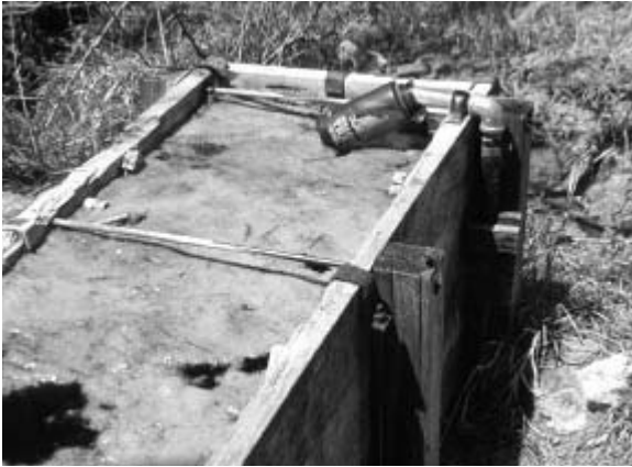
Piped springs can provide clean, fresh water if you take it from the inlet.
