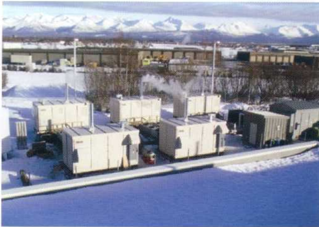
CHAPTER 8, COLOR FIGURE 8.10 Five PC25 power plants provide primary power for a major postal sorting facility in Anchorage, AK. Since beginning operations in 2000, the units have ensured that the facility has never lost power, despite numerous grid disturbances. (Photograph courtesy of UTC Fuel Cells.)
