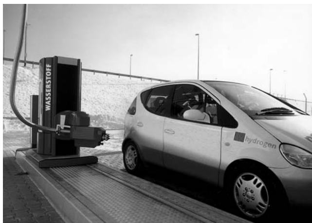
FIGURE 5.4 For the world's first public liquid hydrogen filling station, Linde built the fully automated filling mechanism and supplies the required liquid hydrogen. (Source: www.linde.de .)
