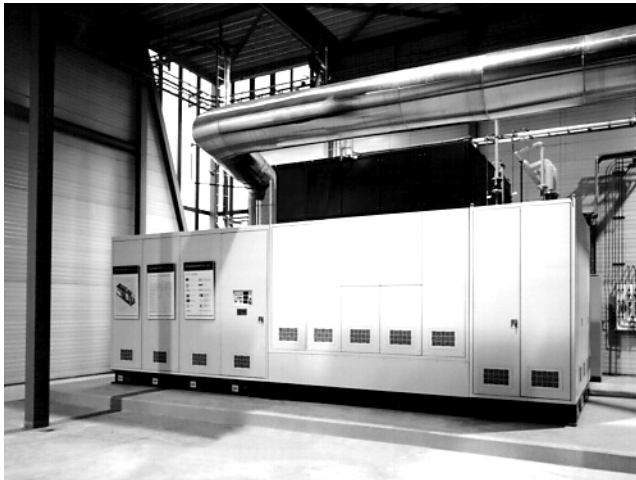
FIGURE 8.13 EDB/ELSAM 100-kW SOFC plant at Westvoort (the Netherlands). After more than 13,000 h of operation, the plant was moved to its new site at Meteorit energy park, Essen (Germany).
