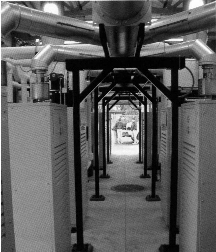
Figure 17-5. Installed Microturbines.
