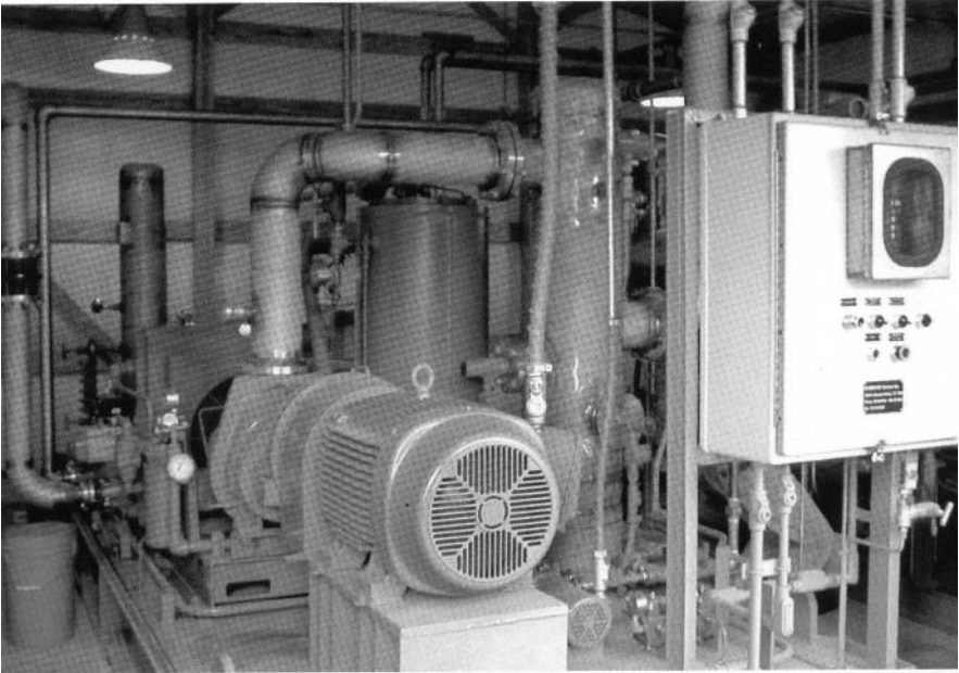
Figure 17-4. Gas Compression System
