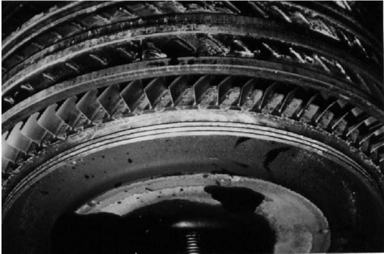
Figure 13-7. View of last stage compressor blades with contamination evident on and between blades. 5,000 horsepower gas turbine-generator unit after 44,500 hours operation.
