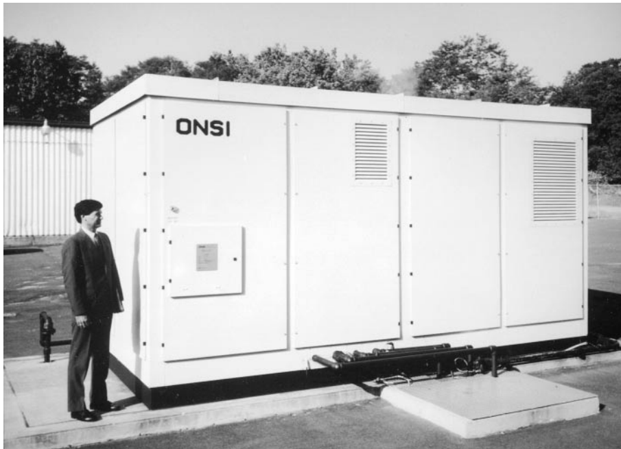
FIG. 27-66 PC-25™ commercial 200-kW PAFC generator. ( International Fuel Cells. )
