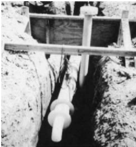
FIGURE B13.96 Example of a low-point leak-detection sump in a plastic gravity drain system.
