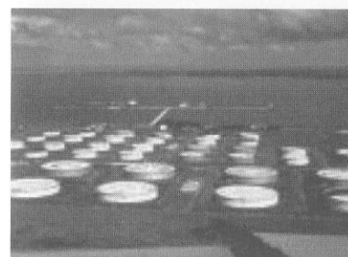
Figure 6-1 Tanks A, B, and C are fixed or floating roof small tanks (less than 10 m diameter) with a total capacity of less than 8000 m 3 ; no intertank spacing requirements other than for construction, operation, and maintenance convenience. Tanks D1 and D2 have diameters greater than 10 m, with the diameter of D2 greater than D1. Intertank spacing between smaller and larger tanks. The photos are of a tank farm and a spherical LPG storage tank. (Courtesy of Red Bag/Bentley Systems, Inc.)
