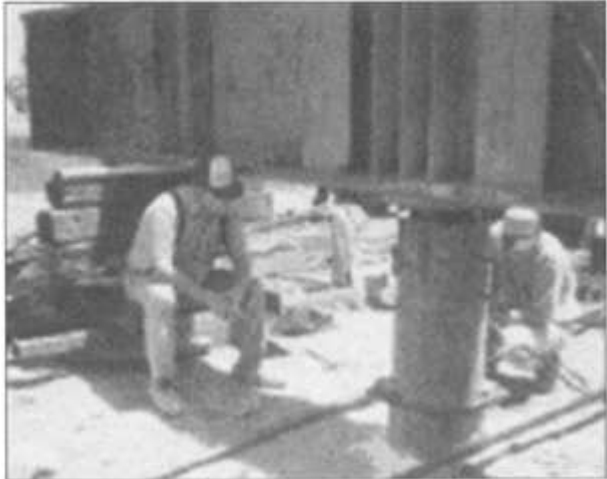
FIGURE 9.21 Pile load testing. (From www.aecigeo.com . With permission.)
