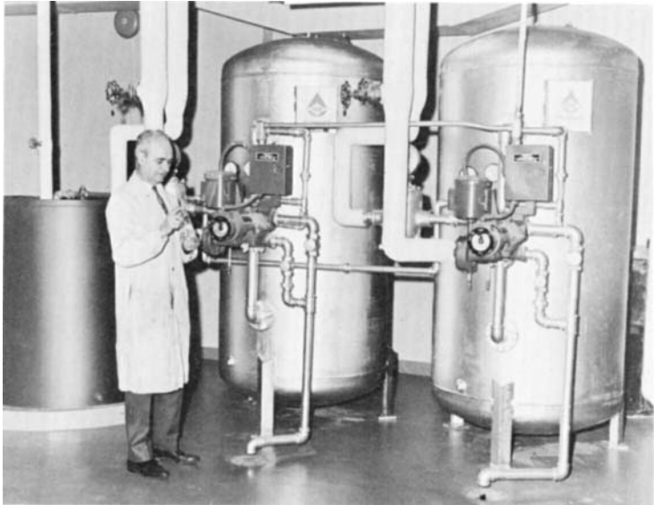
FIG. 12.13 Multiple-unit sodium zeolite installation for continuous delivery of softened water. (Courtesy of The Permutit Company.)
