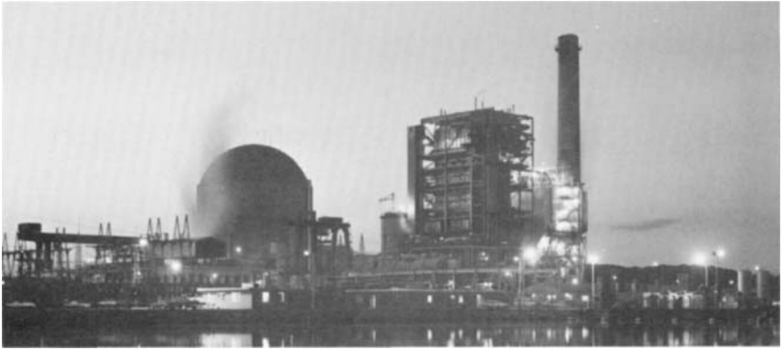
FIG. 34.1 This utility system incorporates both a nuclear unit (left) and a coal-fired unit (right) at the same site. (Courtesy of Carolina Power & Light Company.)
