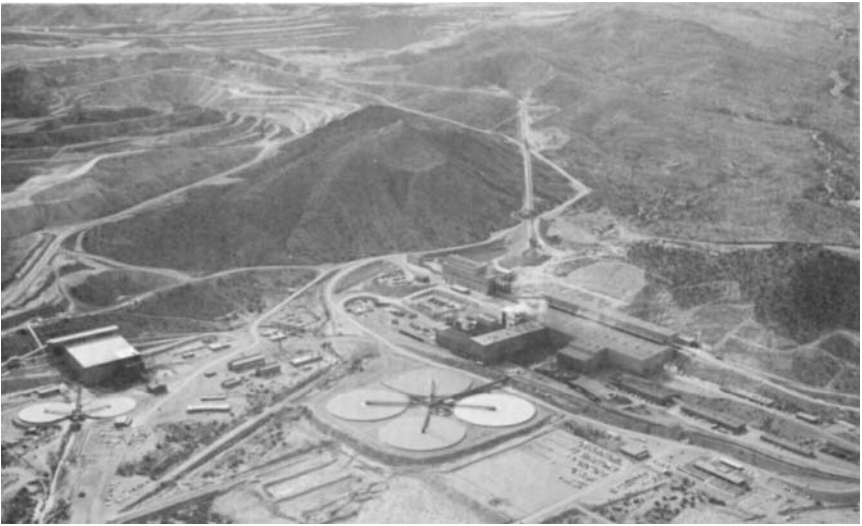
FIG. 29.7 Aerial view of Duval copper-mining operation, Sahuarita, Arizona. (Courtesy of Duval Corporation, Stearns-Roger, Incorporated, and Ray Manley Photography.)
