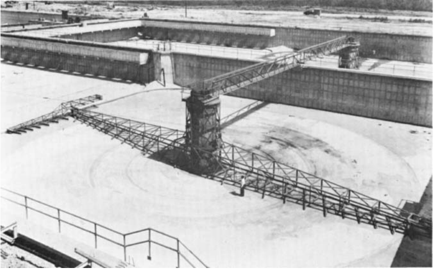
FIG. 9.13 Circular sludge collectors, with rakes designed for corner cleaning. (Courtesy of FMC Corporation.)
