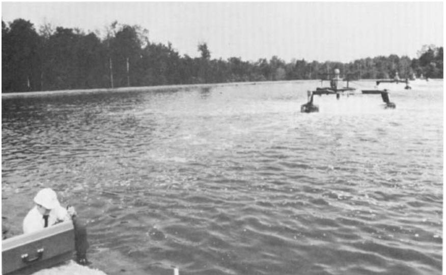
FIG. 23.8 A typical aeration basin works with low F/M ratios and detention times in the 12 to 48 h range.
