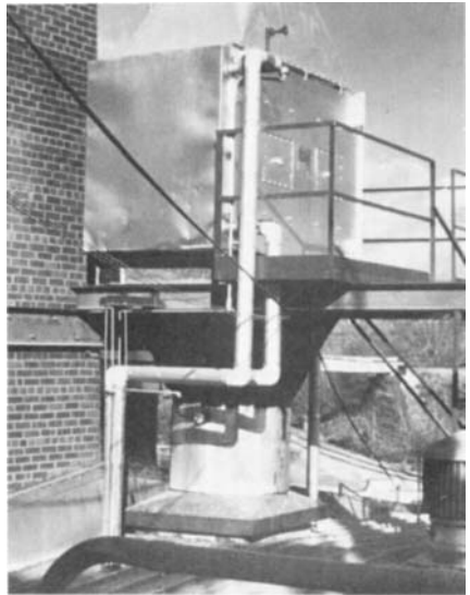
FIG. 39.33 Heat in the stack gases is transferred to feed water in the economizer and also may be recovered by preheating combustion air. The heat-exchange bundle (left) is mounted in the stack (right). (Courtesy of General Resource Corporation.)
