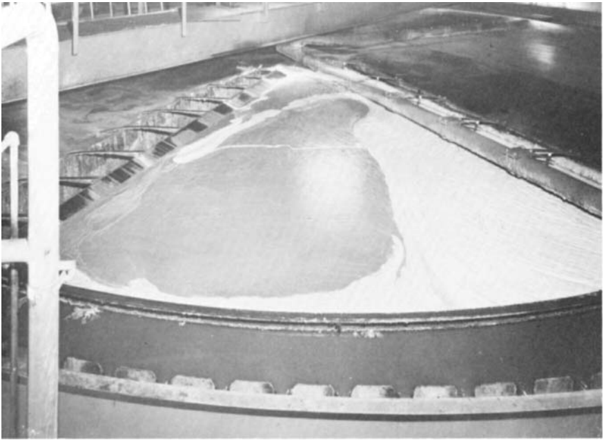
FIG. 11.8 The float produced by dissolved air flotation of an oily wastewater (O/W) emulsion. (Courtesy of Infilco Degremont Incorporated.)
