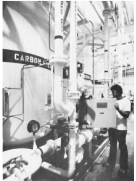
FIG. 17.11 A packaged carbon adsorption system with provision for carbon removal for regeneration at a separate servicing facility. (Courtesy of Calgon Corporation.)
