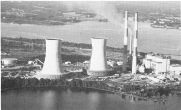
FIG. 38.10 Hyperbolic towers cooling condenser water in a utility station. (Courtesy of The Marley Company.)
