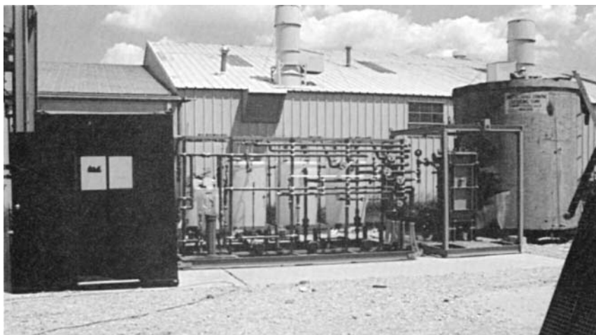
FIG. 40.10 Electro dialysis system processing wastewater for concentration and final disposal. (Courtesy of HPD, Inc., Naperville, Ill.)
