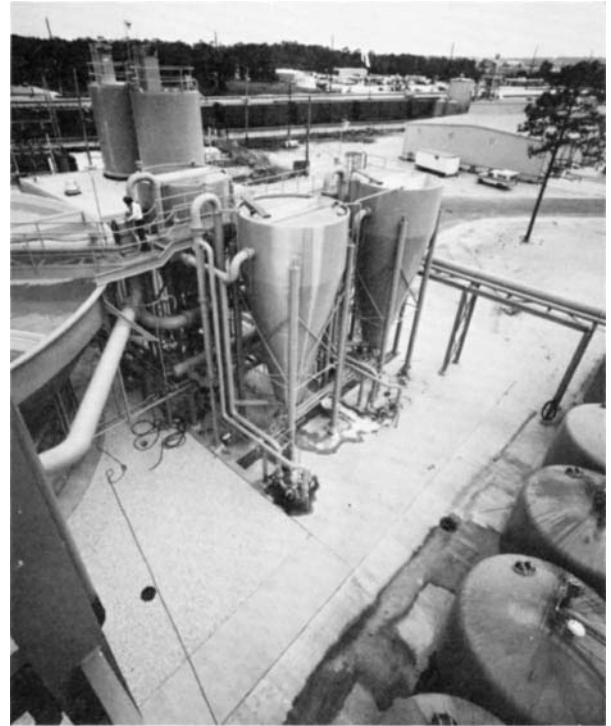
FIG. 10.8 (a) Granular bed lime softener producing a concentrated, pelletlike sludge. (Courtesy of the Permutit Company.) (b) Plant installation. (Courtesy of the Permutit Company.)
