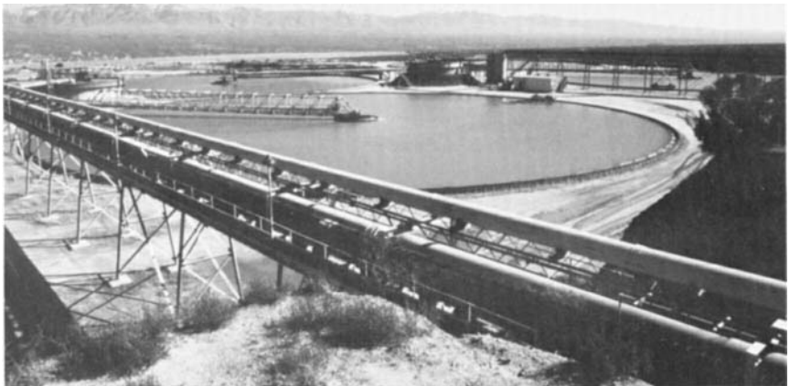
FIG. 29.10 Tailings clarifier-thickeners at a large western copper concentrator.
