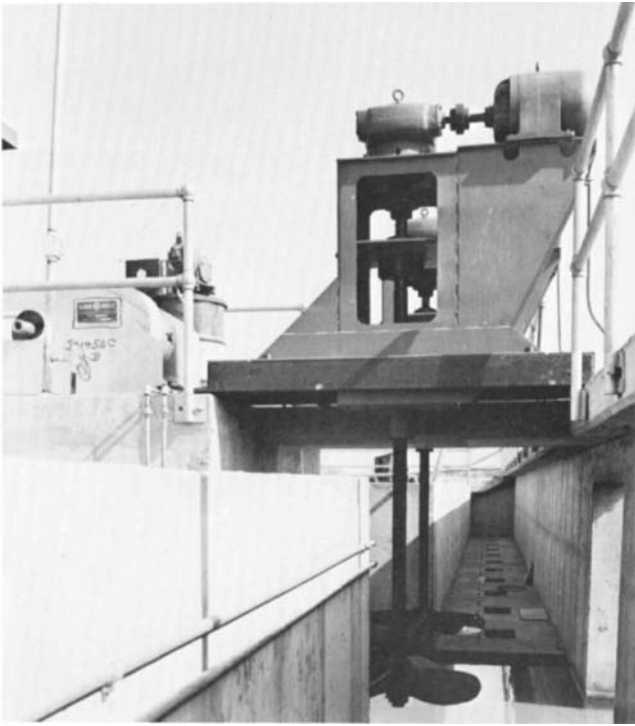
FIG. 8.13 Flash mixers are designed to disperse chemicals throughout the water instantaneously, prior to flocculation. (Courtesy of FMC Corporation, Material Handling Division.)
