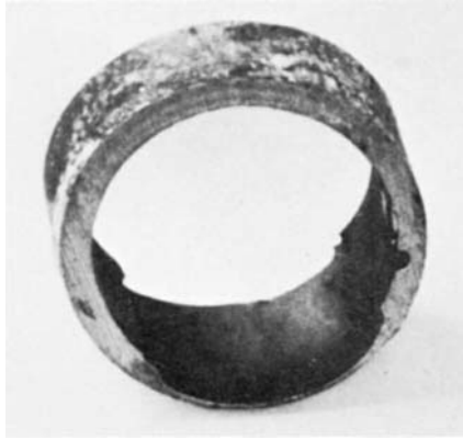
FIG. 39.49 Uniform \text{CO}_2 attack below water line in a condensate pipe.
