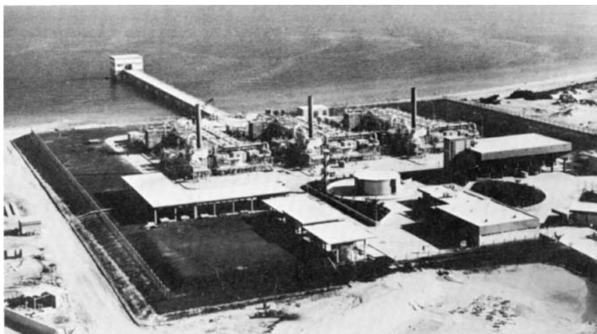
FIG. 18.9 Three flash evaporator modules, each with a capacity of 2.5 mgd (6.7 m 3 /min), producing potable water for Al Khobar, Saudi Arabia. (Courtesy of Aqua-Chem Inc.)
