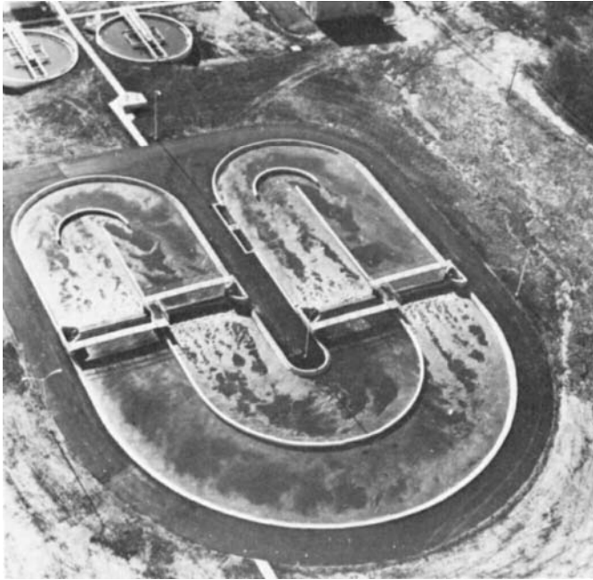
FIG. 23.9 Oxidation ditch processing 2.75 mgd of municipal sewage, with clarifiers in background. (Courtesy Lakeside Engineering.)
