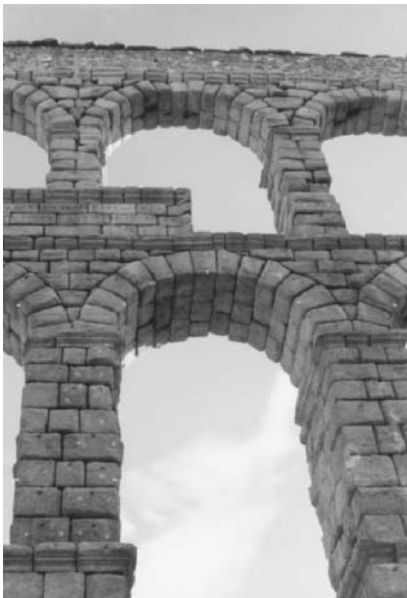
FIGURE 1.32 Two views of the Roman aqueduct bridge in Segovia, Spain. The aqueduct was built on two levels without the use of any mortar or cement. (Photo by Larry W. Mays and copyright by Larry W. Mays)
