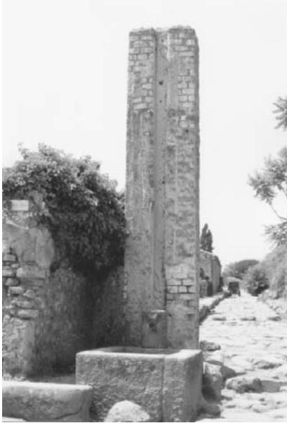
FIGURE 1.46 Brick tower on which secondary castella (lead storage tanks) were mounted on top of the tower. Lead pipes were used for the flow of water to and from the lead tanks and were placed in the vertical recessed portion shown in the tower. The exiting lead pipes ( calices ) branched off to supply individual customers and also supplied the public fountain shown at the base of the tower. (Photo by Larry W. Mays and copyright by Larry W. Mays)
