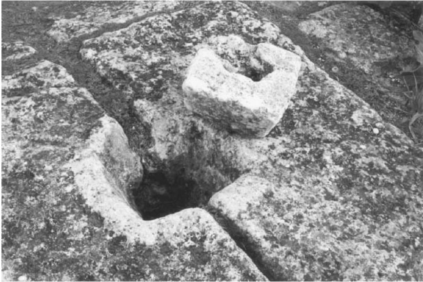
FIGURE 1.20 Cover to underground drainage system for water channel from the Majestic Fountain. (Photo by Larry W. Mays and copyright by Larry W. Mays)
