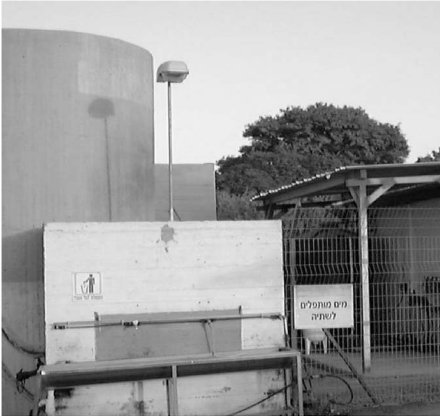
FIGURE 17.10 Desalination of brackish groundwater for drinking water in the village of Ein Yahav in the Arava Rift Valley. (Photograph H. J. Bruins)
