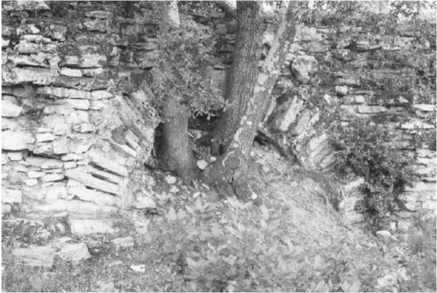
FIGURE 1.28 Aqueduct of Nîmes to the southeast of the Pont du Gard. (Photo by Larry W. Mays and copyright by Larry W. Mays)
