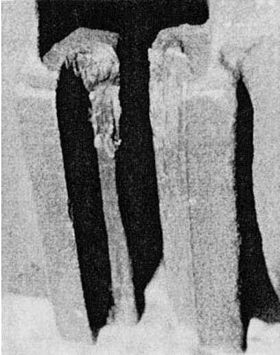
Figure 3-46. Damage to Guide Slots of Flexible Wedge Resulting from Attempted Closure of Wedge Gate Valve with Wedge Rotated and Jammed in Valve Body, Size DN 300 (NPS 12) Class 150. (Courtesy of David Mair.)
